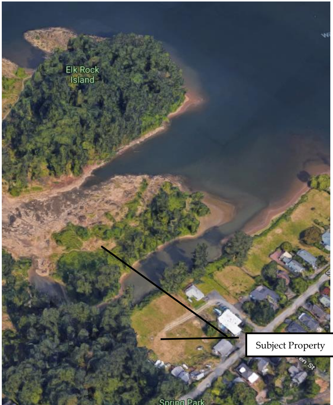
Figure 7. Subject property with the slough and the Willamette River
