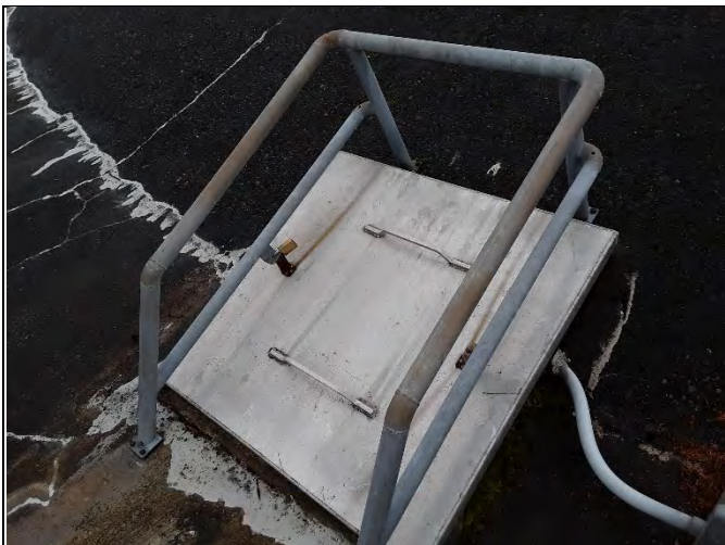
CONCRETE RESERVOIR ROOF ACCESS
