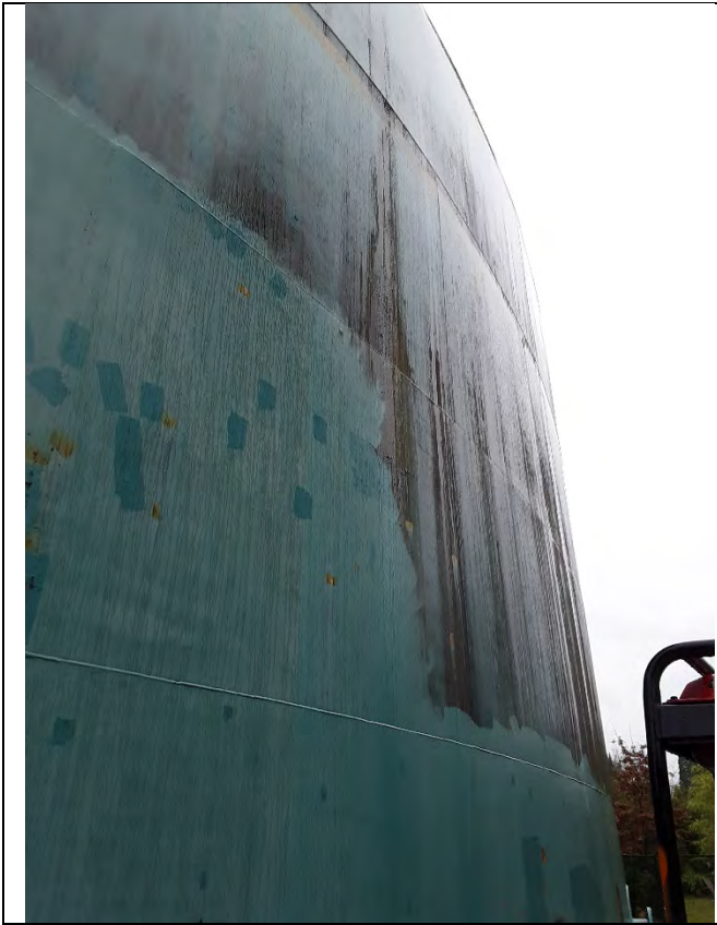
PRESSURE WASHED/UNWASHED SECTION
