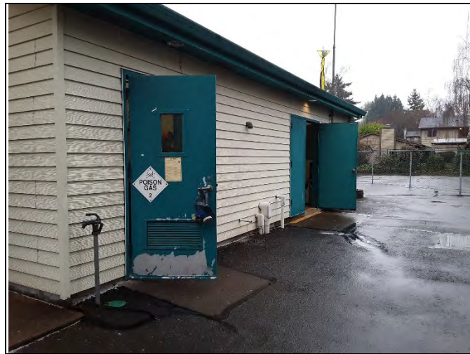
TP47 CHEMICAL ROOM ENTRANCE
