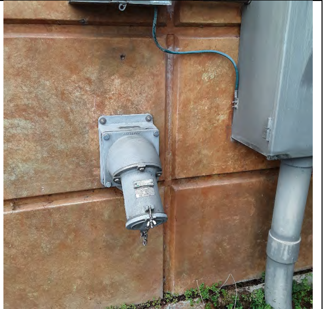
GENERATOR CONNECTION
