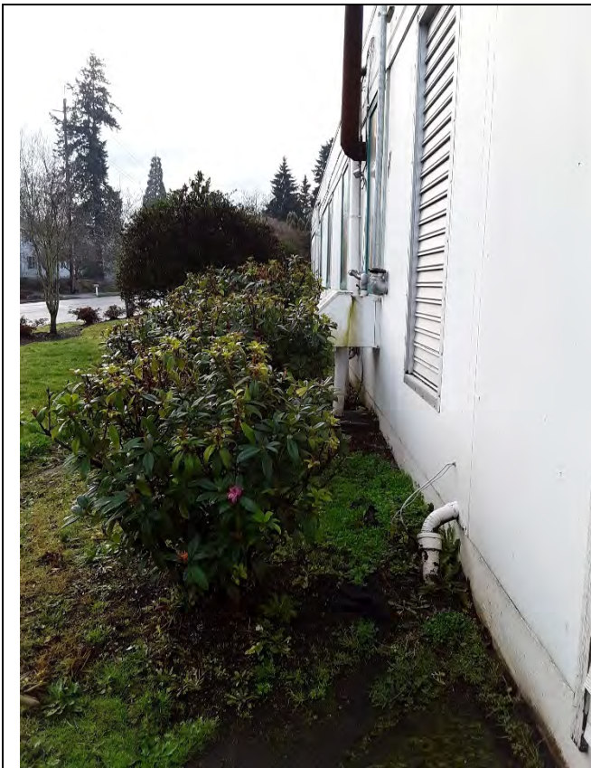
WELL 2 BUILDING EXTERIOR
