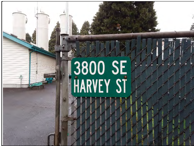
TP235 PERIMETER FENCE
