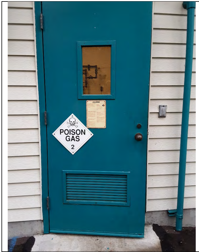
CHEMICAL ROOM ENTRANCE
