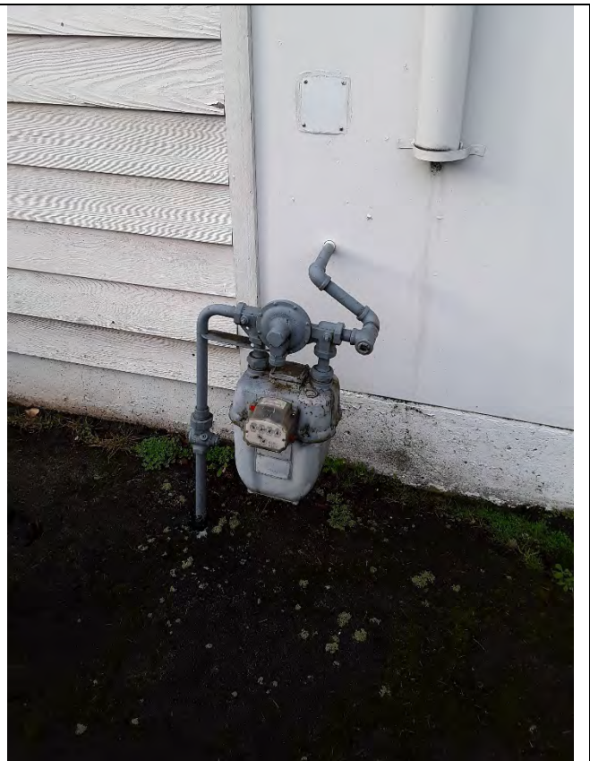
WELL 2 BUILDING EXTERIOR
