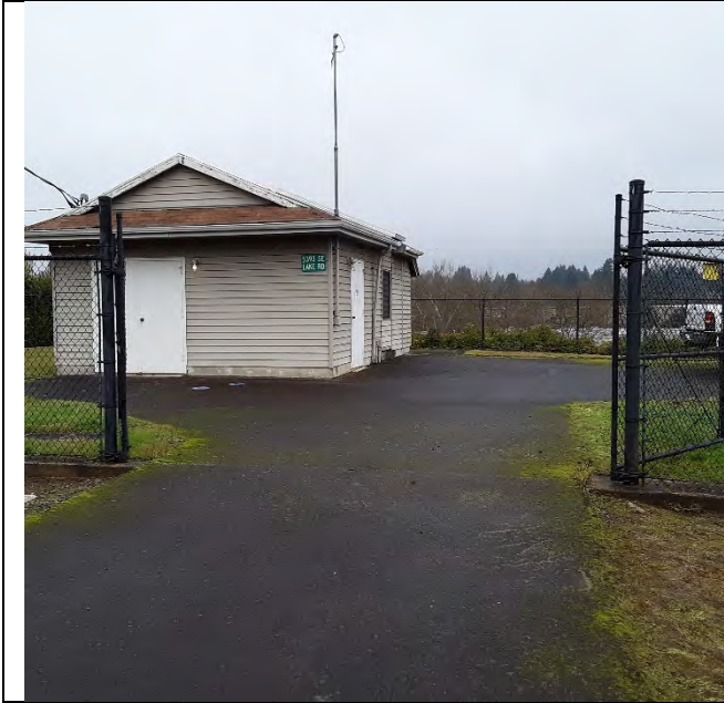
FILTER, GENERATOR & CHEM FEED BUILDING
