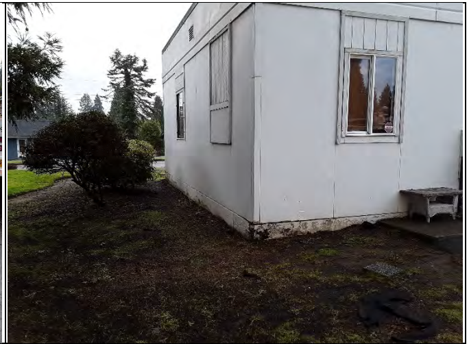
BUILDING EXTERIOR AND SITE
