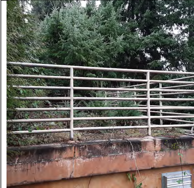
LAVA DRIVE PUMP STATION ROOF
