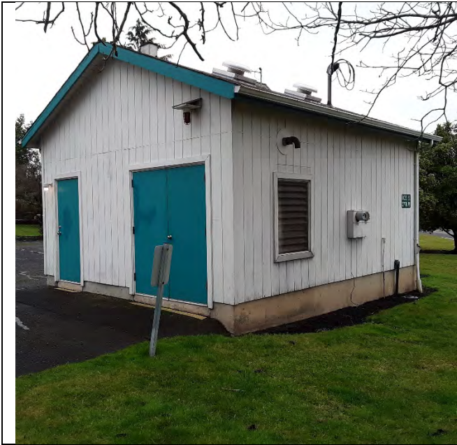
WELL NO. 6 PUMPHOUSE
