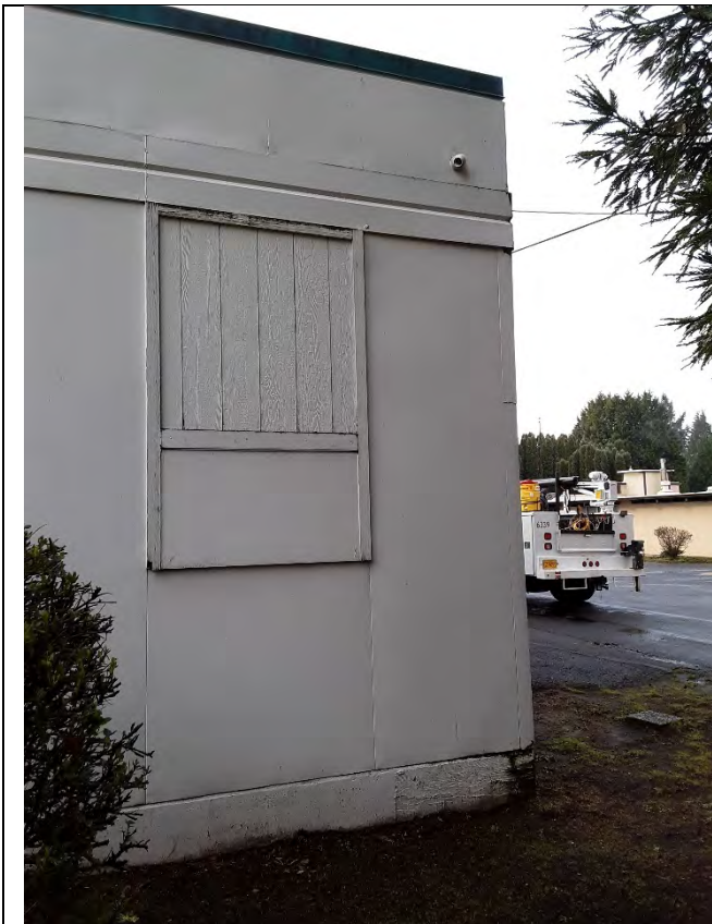
WELL 2 BUILDING EXTERIOR
