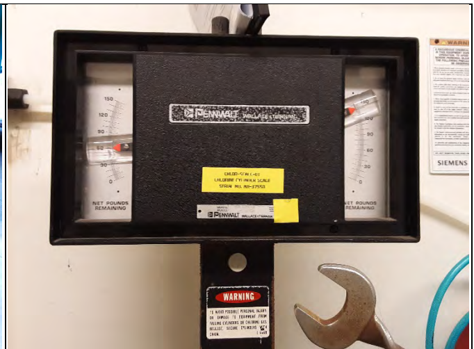
TP235 CHLORINE SCALE
