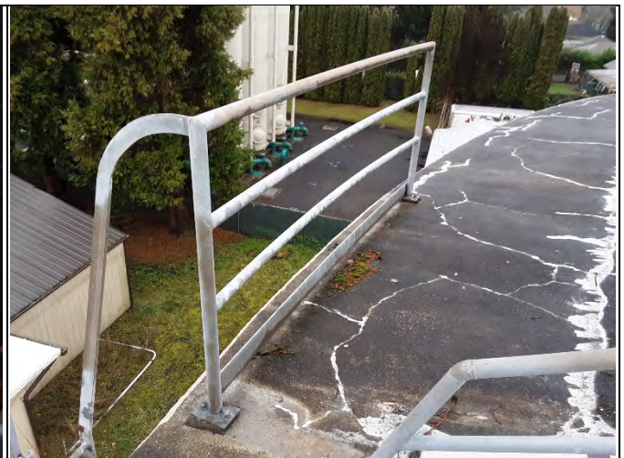
CONCRETE RESERVOIR ROOF
