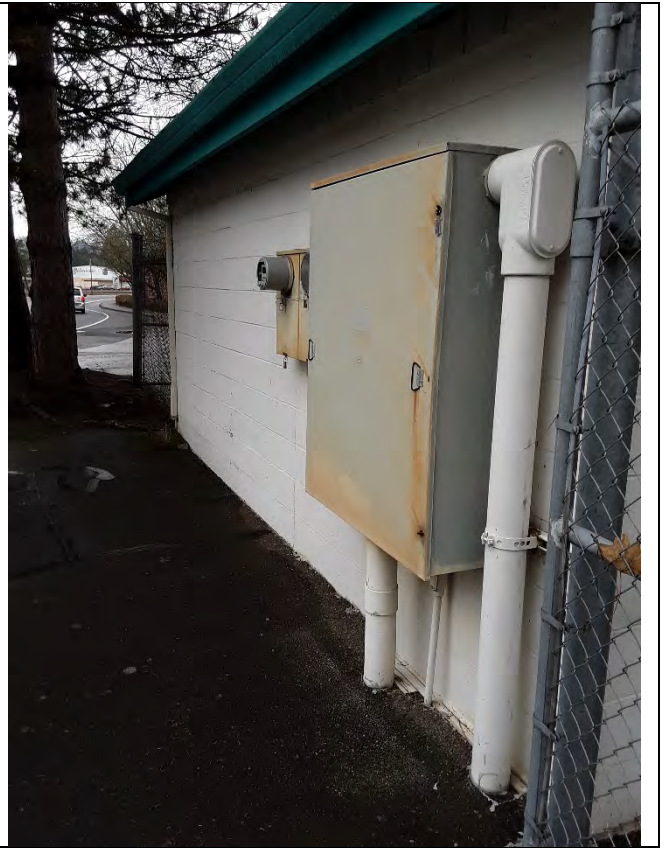
WELL 4 BUILDING EXTERIOR
