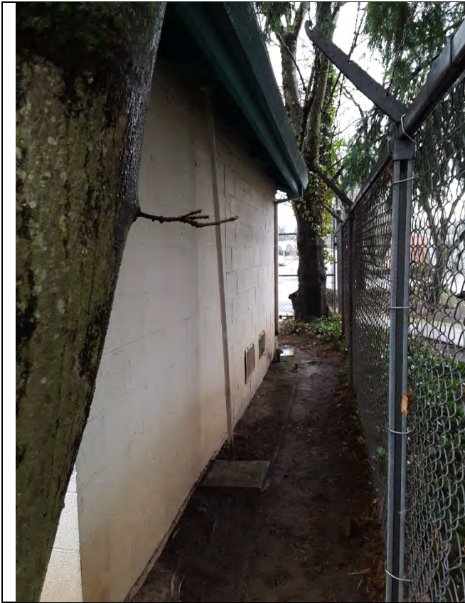
WELL 4 BUILDING EXTERIOR & PERIMETER FENCE
