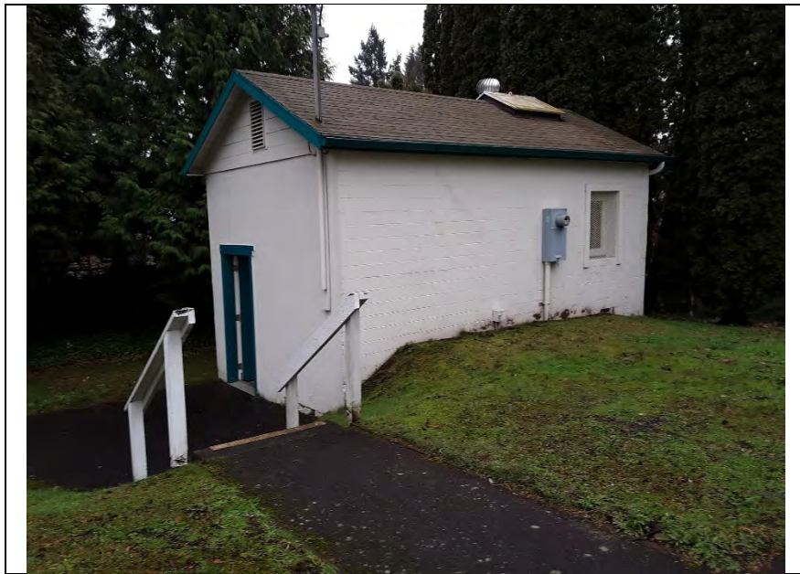
WELL 3 PUMP HOUSE
