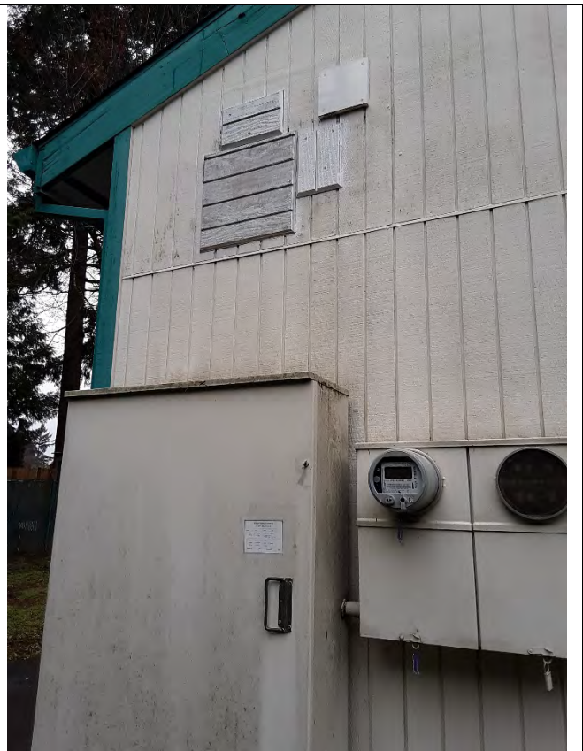
BUILDING EXTERIOR – REPAIRED SIDING
