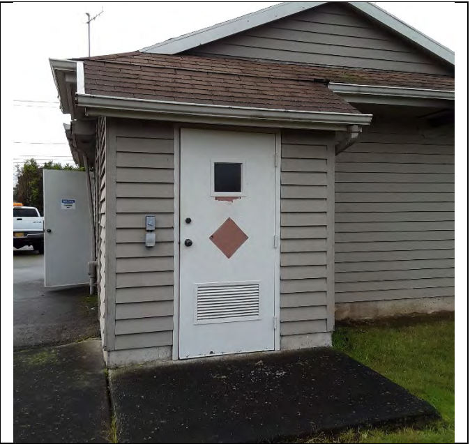
CHEMICAL FEED ROOM ENTRY
