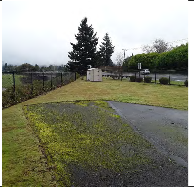
WELL NO. 8 PUMPHOUSE
