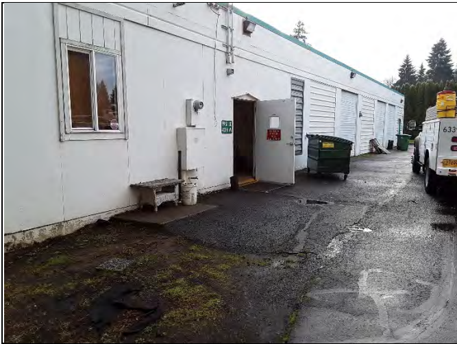
BUILDING EXTERIOR AND SITE
