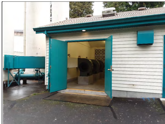
TP235 BLOWER ROOM ENTRANCE
