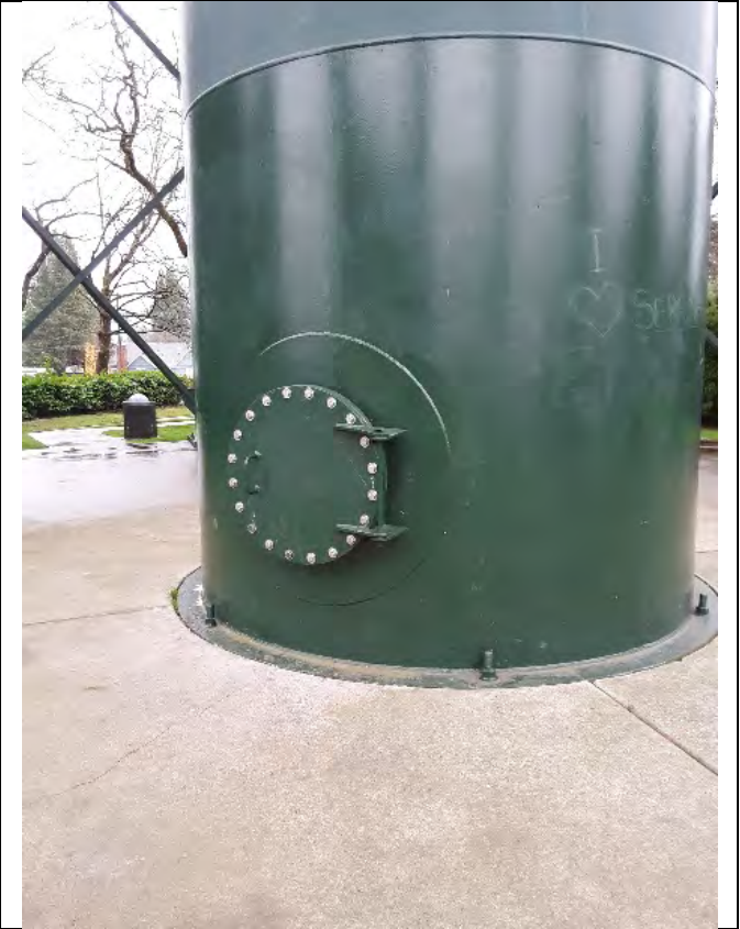
ELEVATED RESERVOIR – HATCH OPENING
