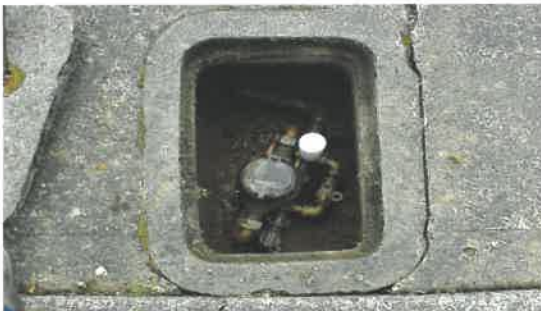
#93-WM sample station typical installations
