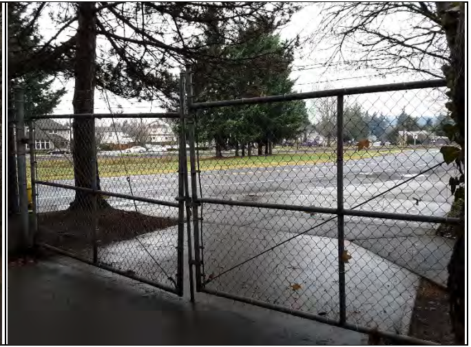
WELL 4 PERIMETER FENCE
