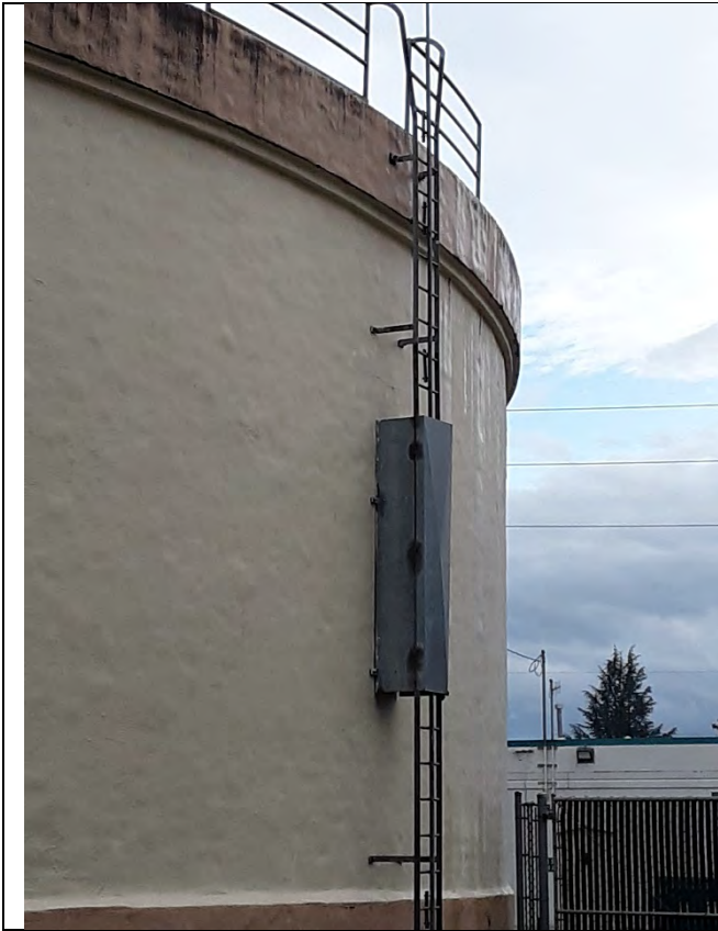
CONCRETE RESERVOIR LADDER
