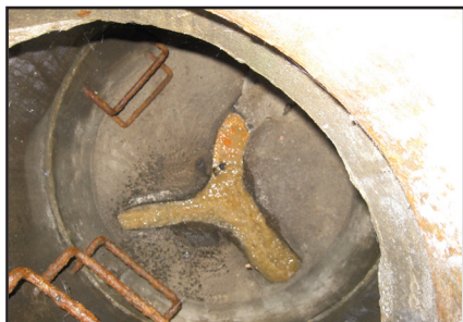
Grease clog in sewer
