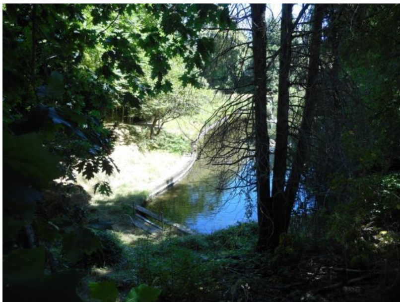
Site location: 002 Photo number: 017 Description: Concrete impoundment at Mill site.
