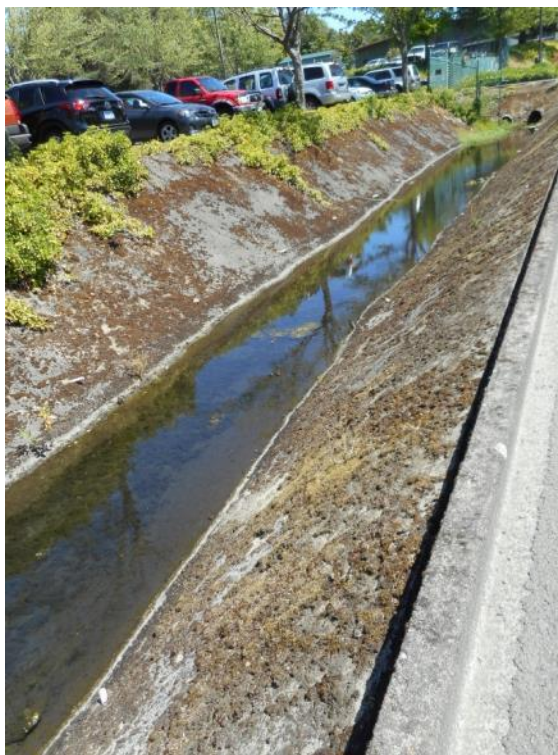
Site location: 005 Photo number: 032 Description: Concrete lined portion of channel.
