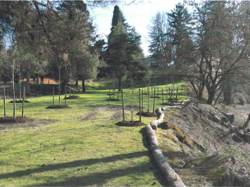
Straw wattles for erosion control
