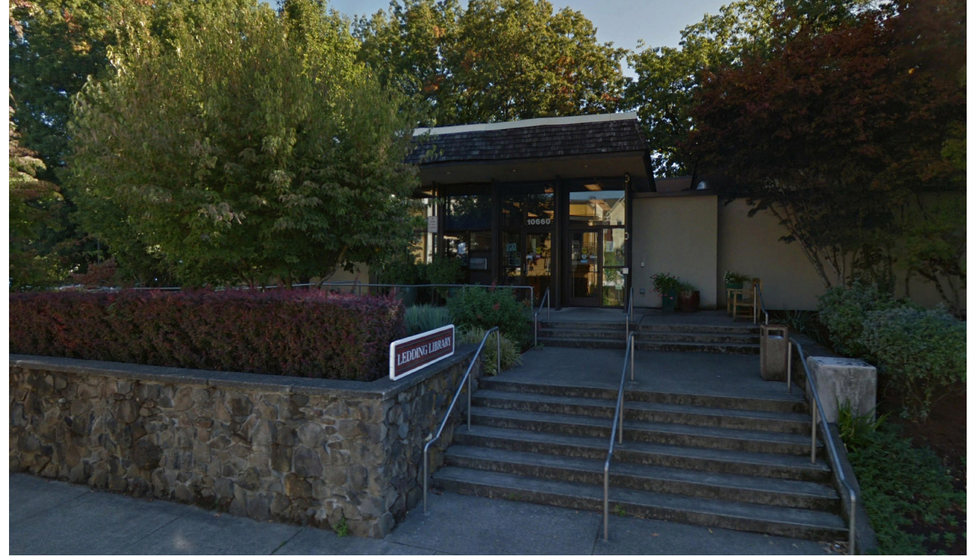
EXISTING STREET VIEW 4 - LOOKING NORTH TOWARD THE EXISTING LEDDING LIBRARY ENTRANCE
