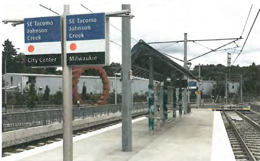
Tacoma Light Rail Station
