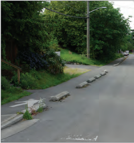
Wheel stops provide physical separation for pedestrians and delineate the travel way.
