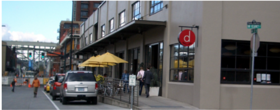
Figure Xc. Retrofitted industrial building with horizontal awnings.
