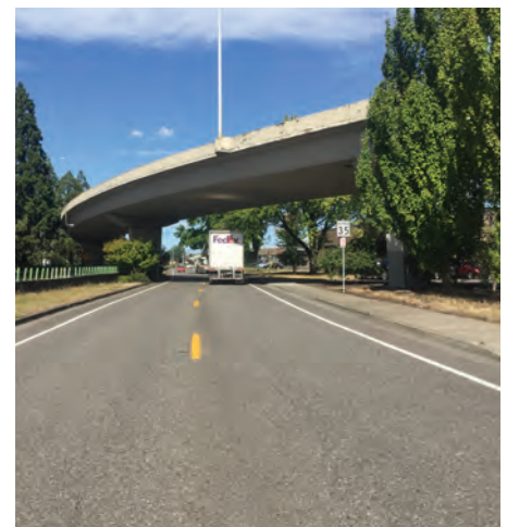
McLoughlin Boulevard and Highway 224
