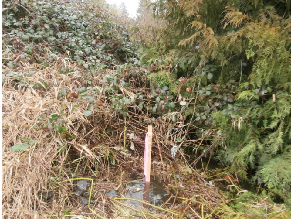
Photo G. View west of stream prior to blackberry being cleared, showing stagnant water at potentially blocked inlet to culvert under SE 37th Avenue.
