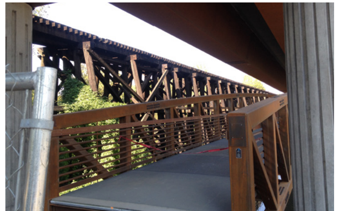
TriMet pedestrian bridge at north end of the site
