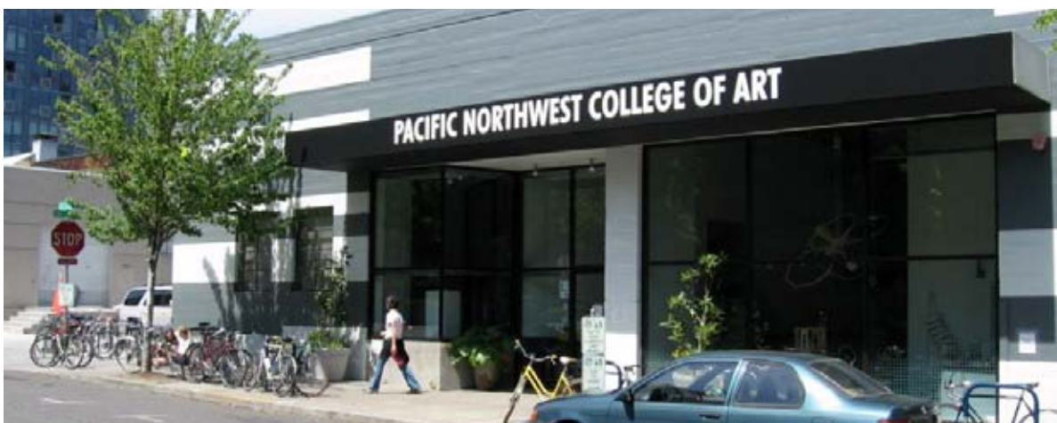
Figure 8. Retrofitting Industrial Buildings with Horizontal Awnings
