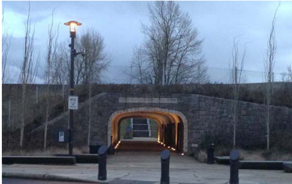
Figure 26. Example of pedestrian undercrossing, Washougal, WA.
