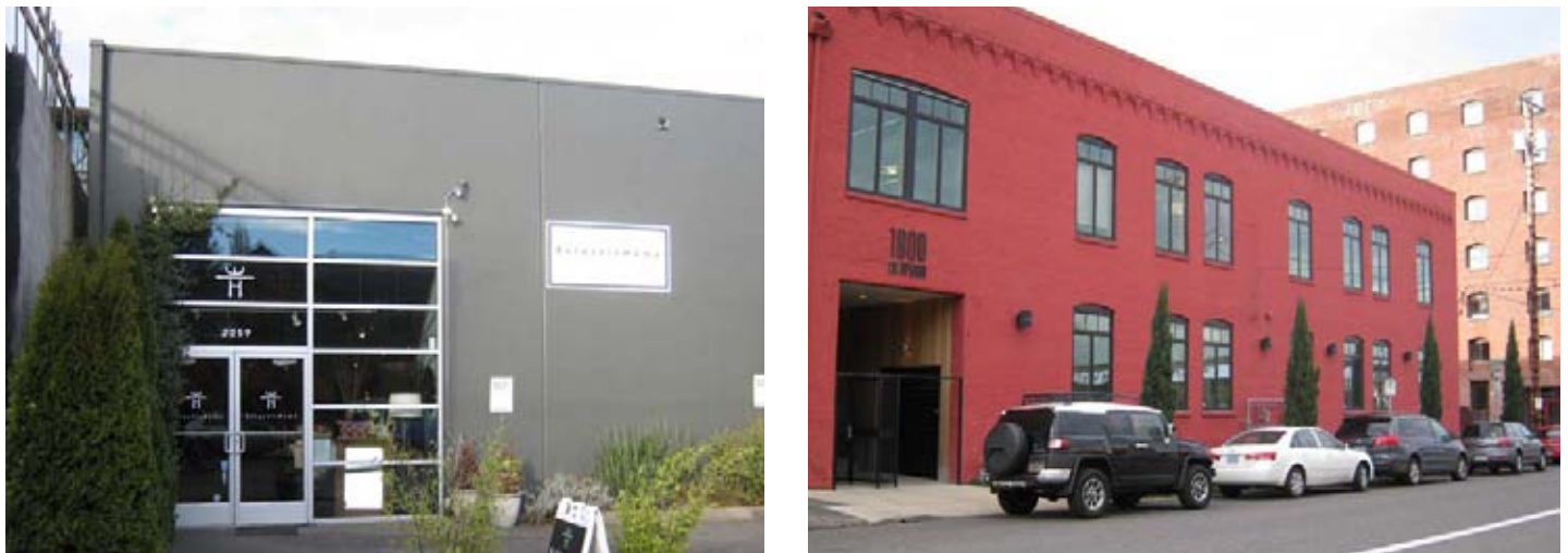
Figure 13. Examples of façade improvements to existing industrial uses
