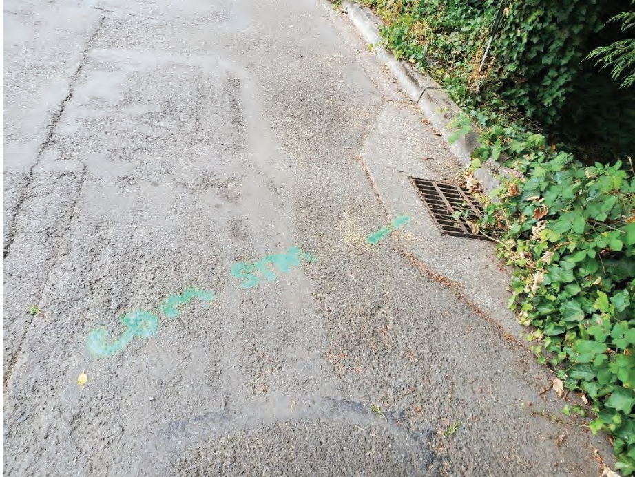
Photo 5 . Stormwater drain sends water to the stormwater ditch. The is one of two sources, the other is piped from the Lynwood Elementary School and possibly other more distant developments.
