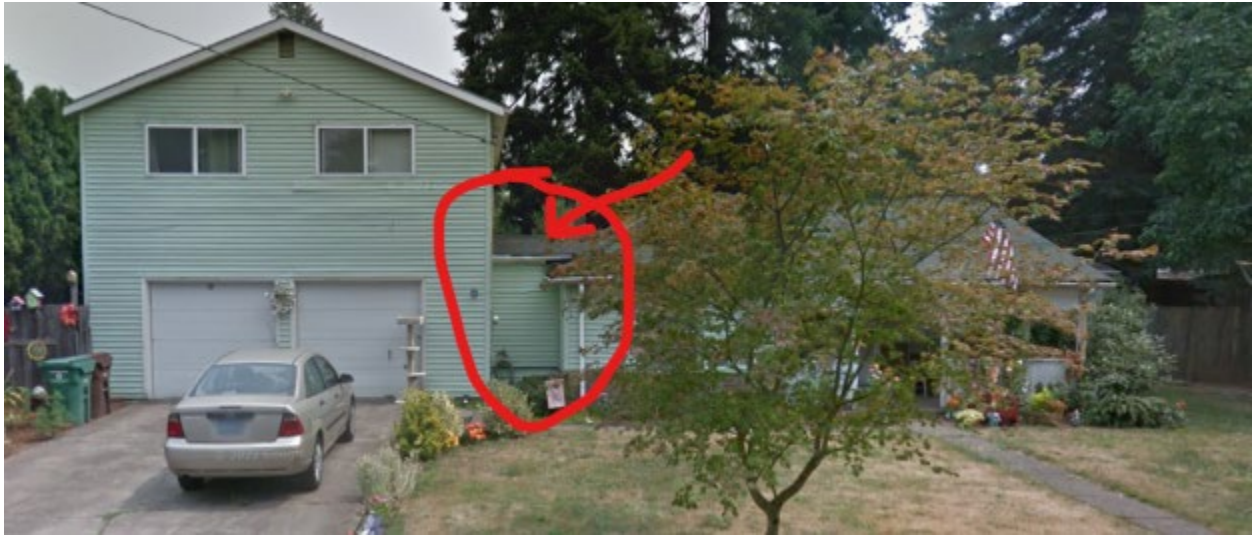
The red circle is drawn around the enclosed breezeway propped to be removed.
