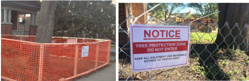
Above: Examples of tree protection practices
