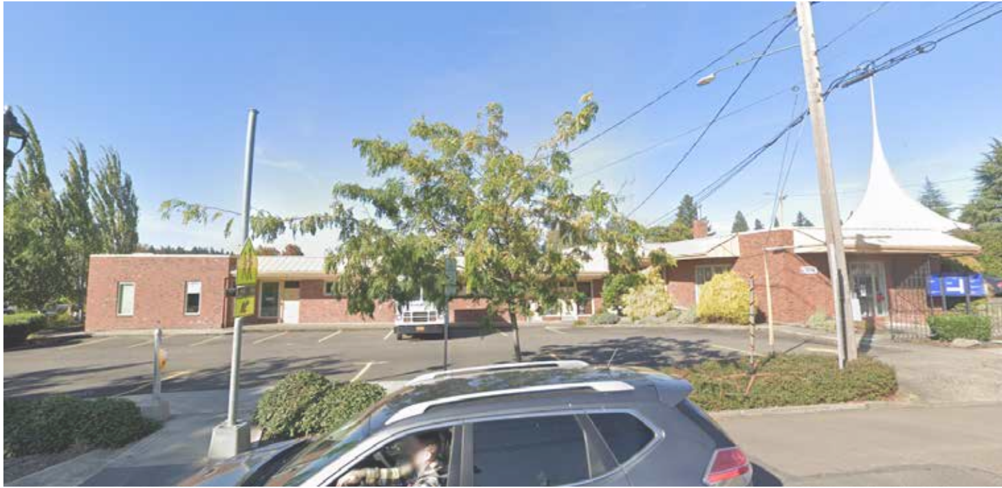
Commercial Complex, View looking North from the intersection of SE Washington & SE 23rd
