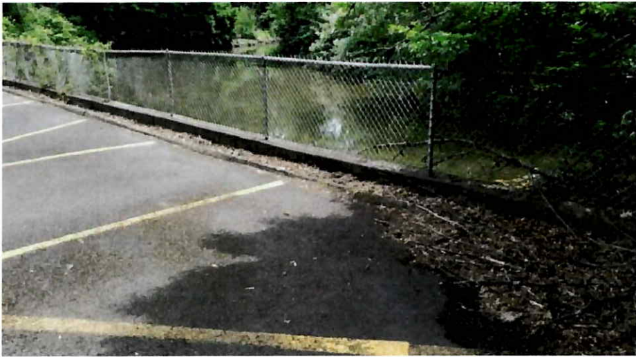
Photo A. View facing southerly of the on-site paved VC and the off-site Primary Protected Water Feature (pond) in the background.
