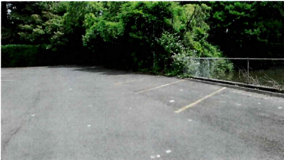
Photo C. View of existing paved on-site VC associated with off-site pond.
