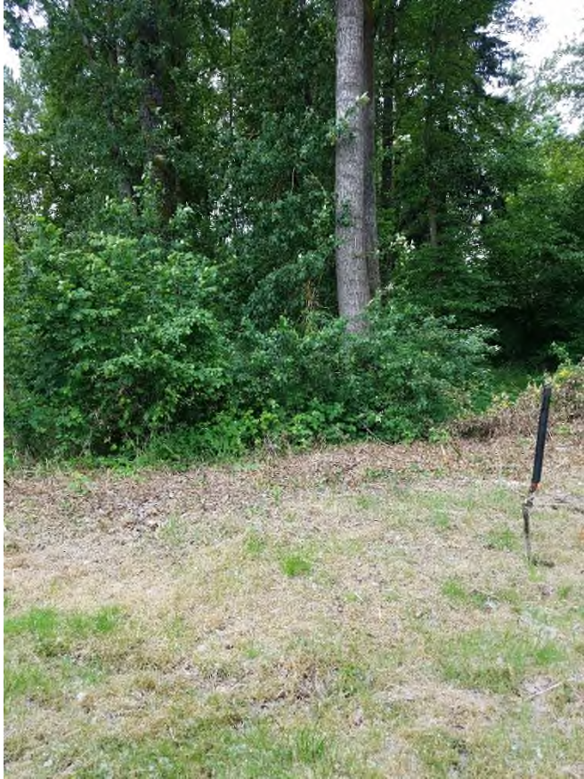
Photo 9. The border between the Sparrow ROW and property line. The north side of the channel slope showed signs of having fill material. ETC Photo 5/25/18.
