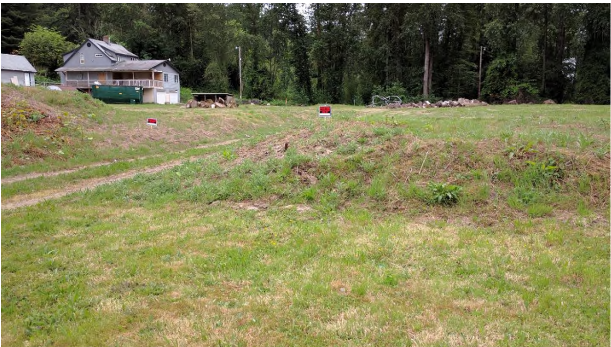
Photo 2: A clear view of the fill that is the study area. The house is 12225 SE 19 th Avenue. ETC Photo 5/25/2018
