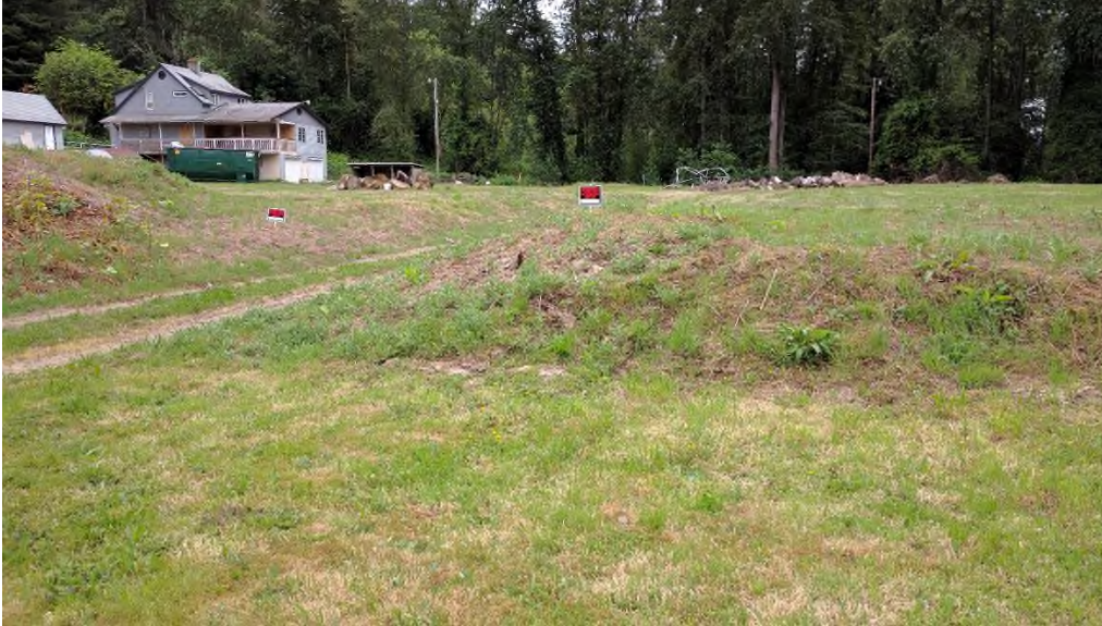
Photo 1. A view of the subject property looking from north to south onto the property, we believe we are looking at the amount of fill that is on the property. The road through the middle of the property is also visible. ETC Photo 5/25/2018
