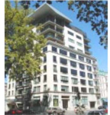
Recommended: Contemporary additions on rooftops can be compatible with the historic building if the historic facades are left intact (NW 8th and Everett, Portland)
