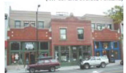
Recommended: Addition of second story building is set back from the historic facade (Boulder, CO)
