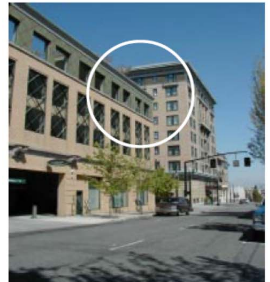
Recommended: Basic proportions, silhouette and distinctive elements of the historic hotel were repeated in new adjacent parking structure (SW 16th and Yamhill, Portland)
