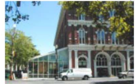
Not Recommended: Addition does not relate well in form, massing or materials (SW 2nd and Ankeny, Portland)
