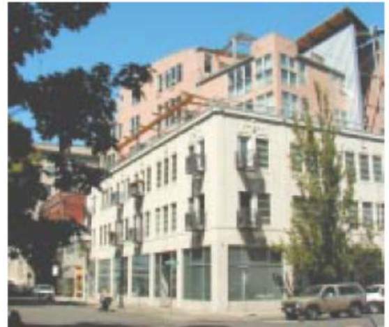
Not Recommended: Contemporary addition on top of historic building contrasts too greatly in form, color and materials with the existing building below. (NW 8th and Flanders, Portland)
