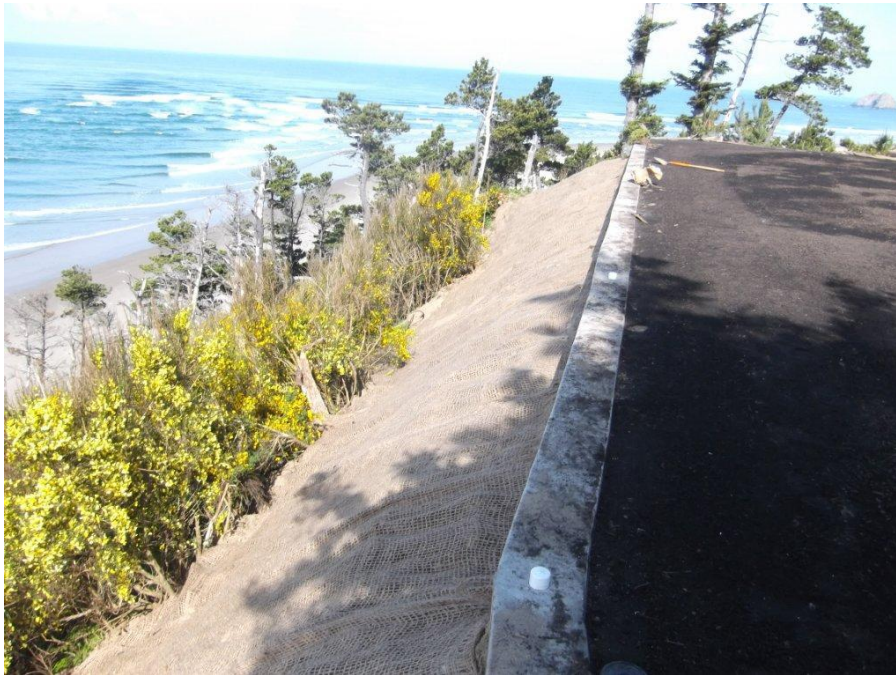
Photo 3: Micropile wall after slope reconstruction. Vegetation has not yet been installed.
