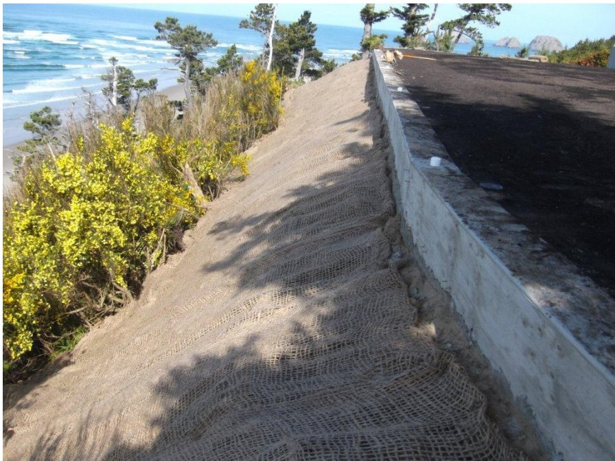
Photo 2: Micropile wall installed. Slope has not been reconstructed.
