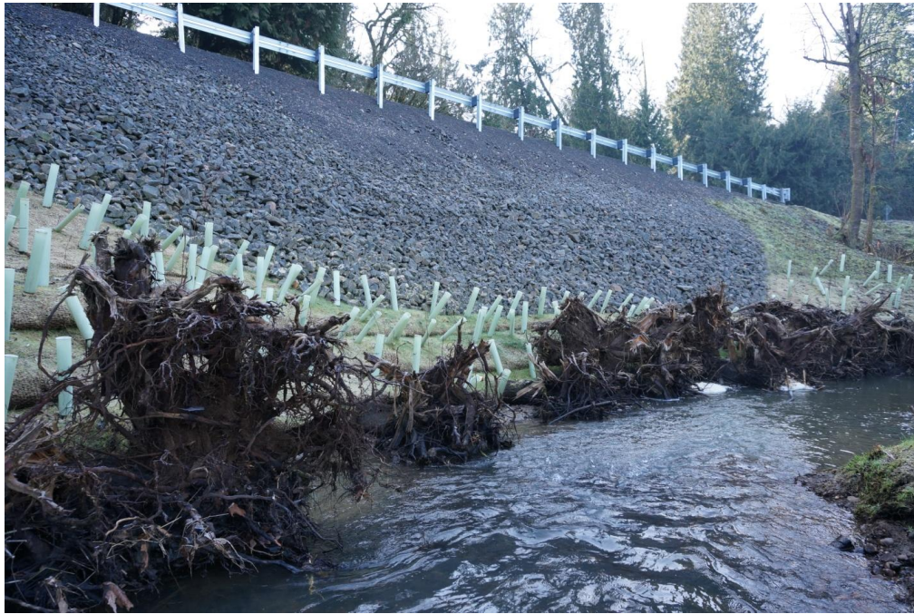
Photo 4: Rock slope stabilization with logs and planting at toe in Clark County, WA. The blue tubes are browse protection for the installed plants.
