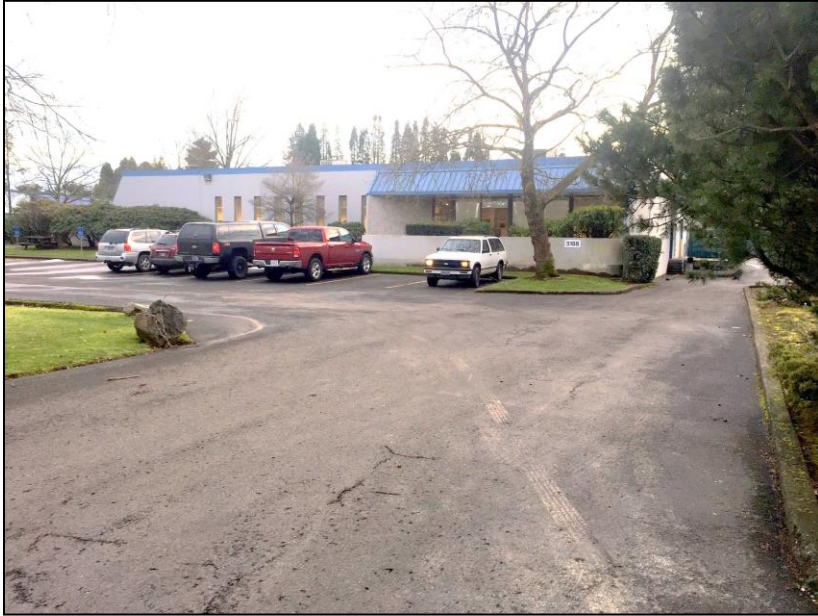
HVAC – property adjacent to BRM to the southeast.
