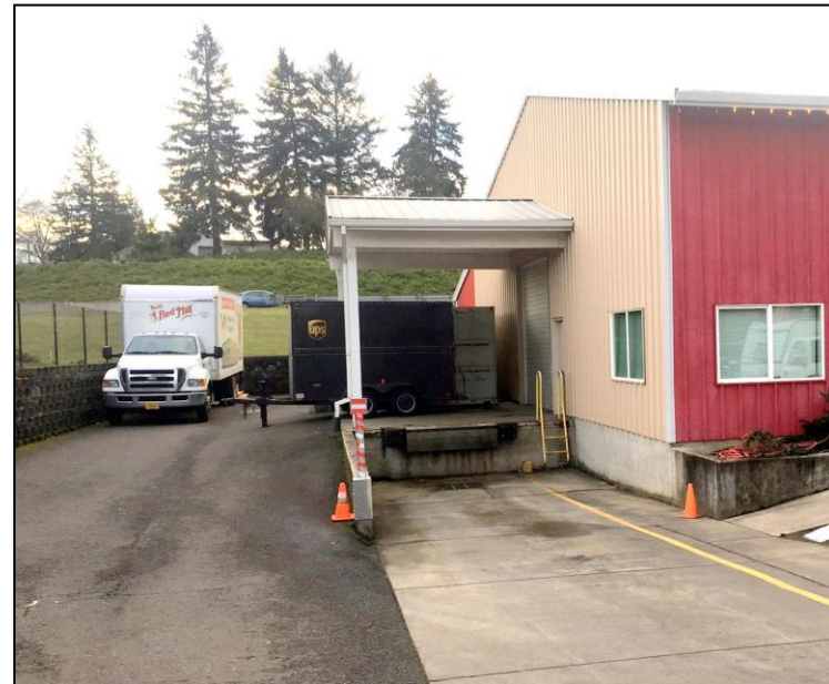
Warehouse loading dock. The truck is parked in proposed sign location. Note elevation of Hwy 224 roadway is at roof of truck.
