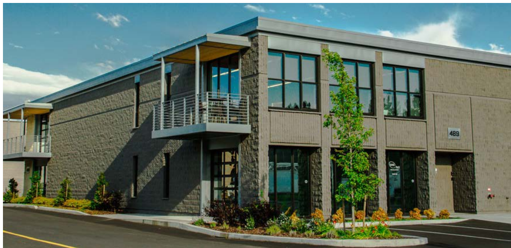
Figure 6. Example of ground floor windows
