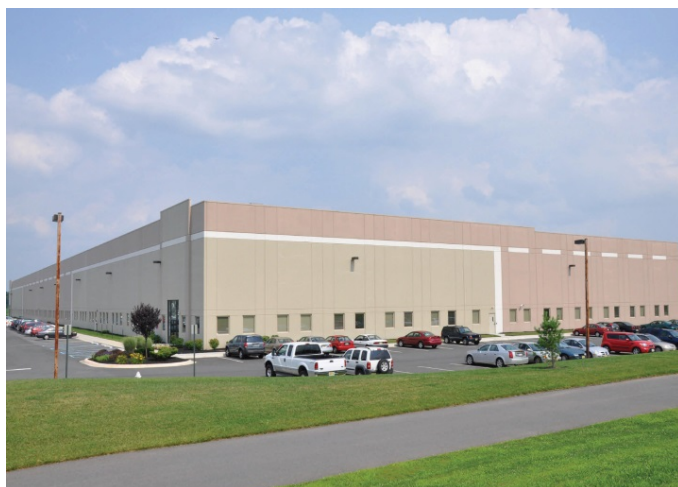
Source: Dolan Contractors, Inc., Westampton, NJ
