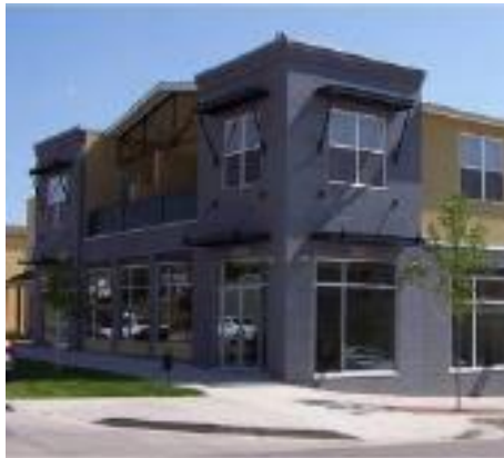
A Light Industrial Flex building that addresses the street with windows and front entrances, awnings and interesting architectural detailing. This building type supports manufacturing, office and retail uses. Source: City of Denver, CO
