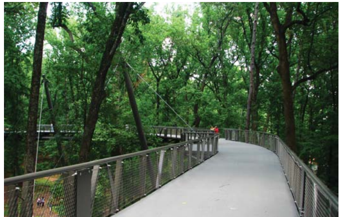
Example of a multi-use pathway, elevated through south forest area
