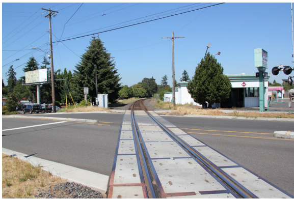
The railroad crossing at SE Harrison St requires improvements to increase pedestrian safety.
