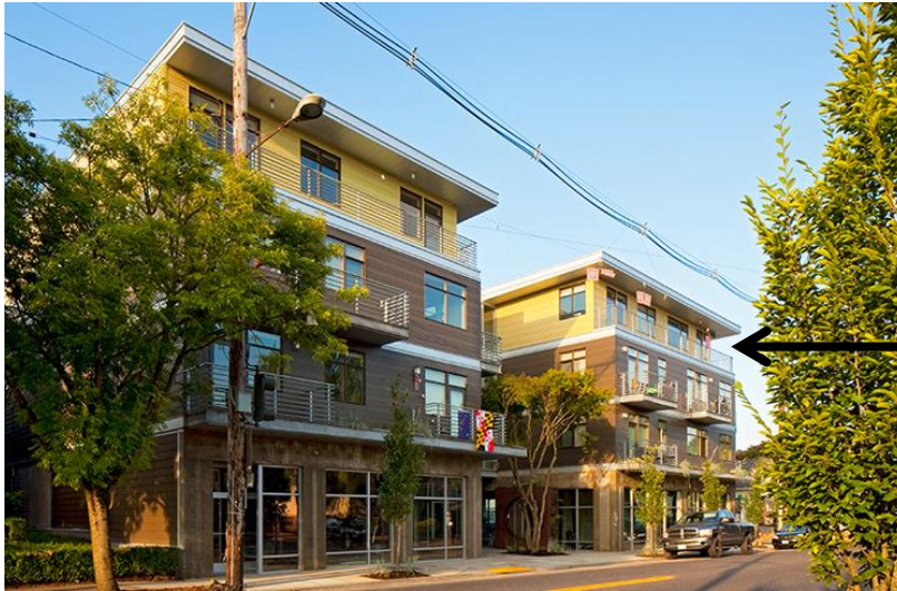
Figure 5. Example of a building step back (3810 SE Division St)
