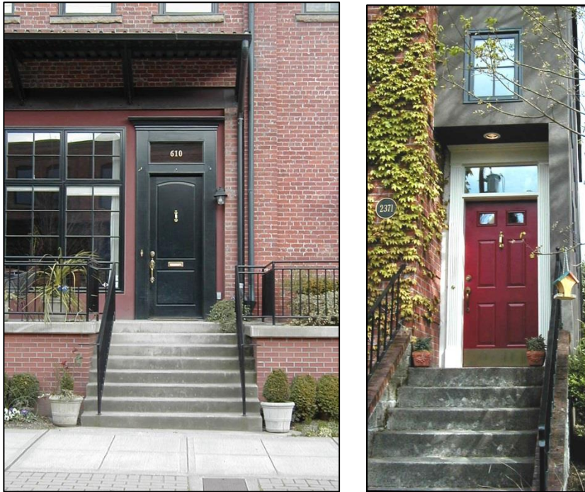
Figure 10. Transition area provided by a grade separation and patio (left) and a grad separation (right).
