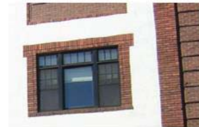
Stucco and brick
