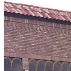
Terra cotta and brick
