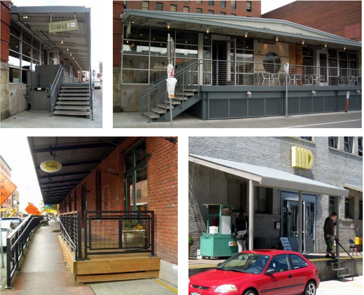
Figure 9. Incorporating existing elements such as loading docks and covered bays can help retain the area's unique character
