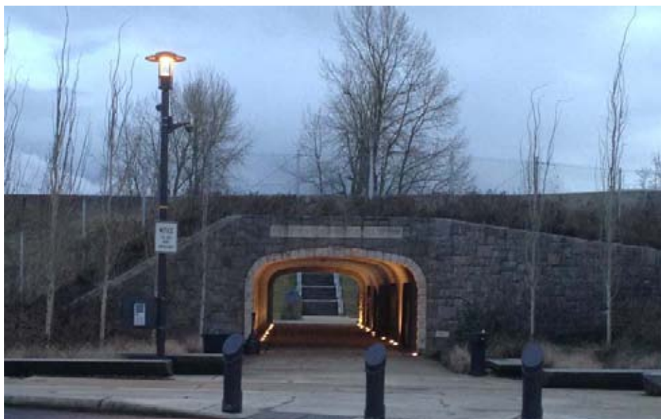
Figure 26. Example of pedestrian undercrossing, Washougal, WA.
