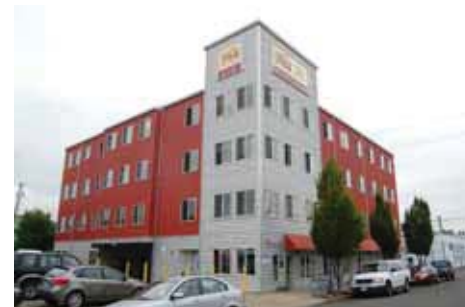
Figure 7. This new employment incubator project within the Central Eastside Industrial District provides affordable office and artist space. The building illustrates how new development can relate to the surrounding industrial character by using “industrial” building materials, and also demonstrates how buildings can provide architectural elements to address the corner.
