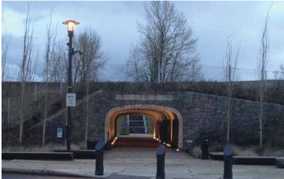
Figure 18. Example of pedestrian undercrossing, Washougal, WA.
