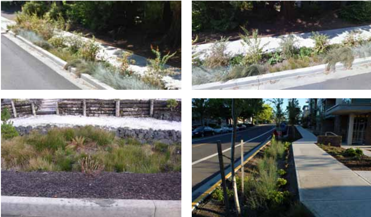
Figure A-7. Examples of linear stormwater swales, as proposed for Local Streets
