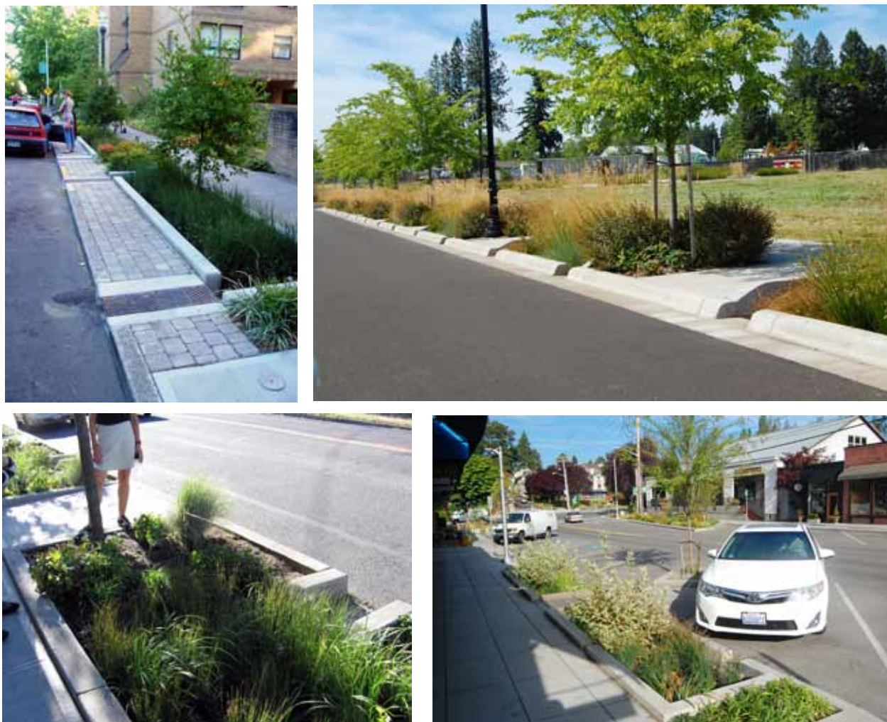
Figure A-6. Examples of constructed stormwater planters, as proposed for key streets
