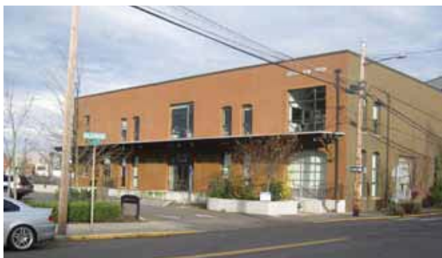
Figure 19. Industrial development with no setback from the sidewalk and parking lot landscaping.
