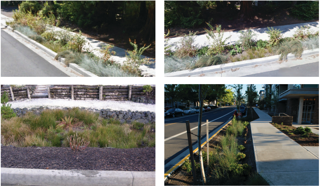
Figure 6. Examples of linear stormwater swales, as proposed for Local Streets
