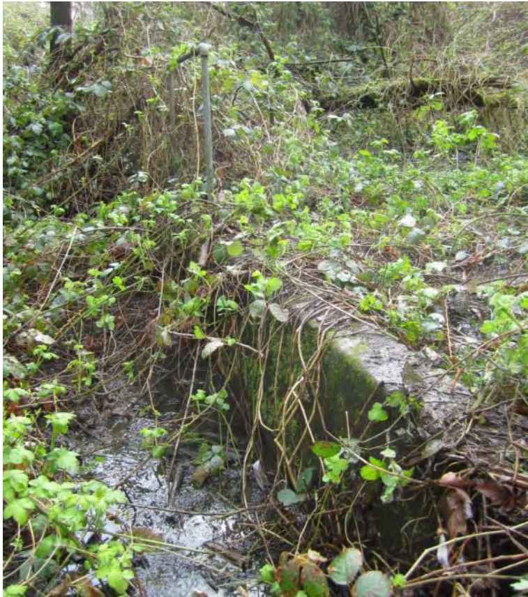
Photo 4. The remnant concrete wall.
