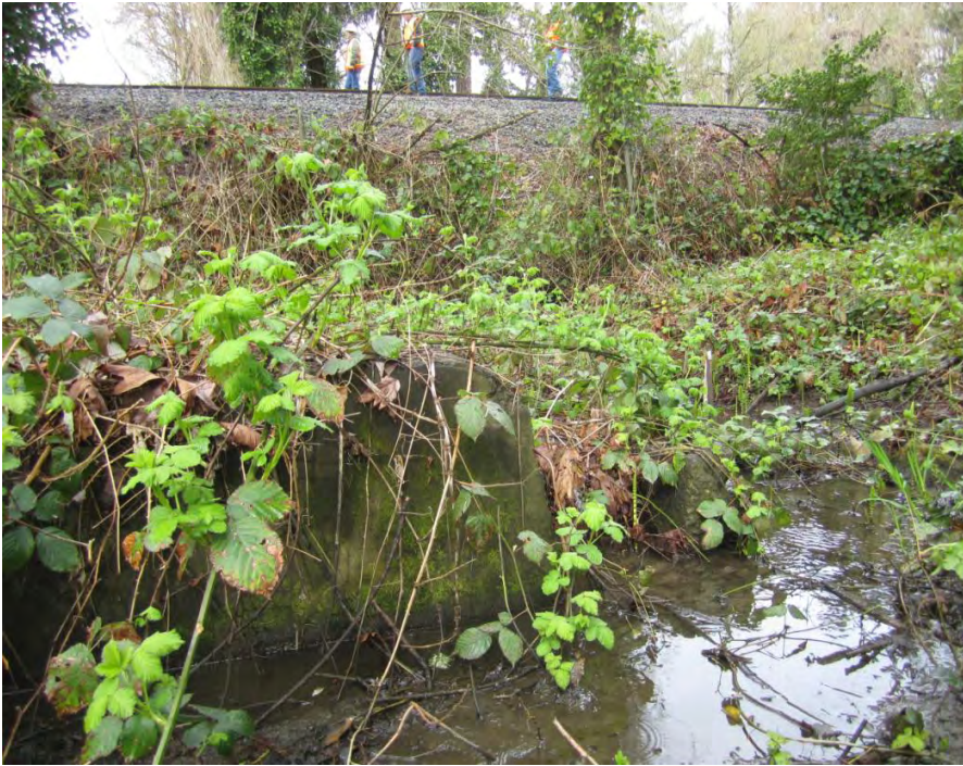
Photo 3. Concrete wall that spans Crystal Creek and intercepts and diverts flow from channel.
