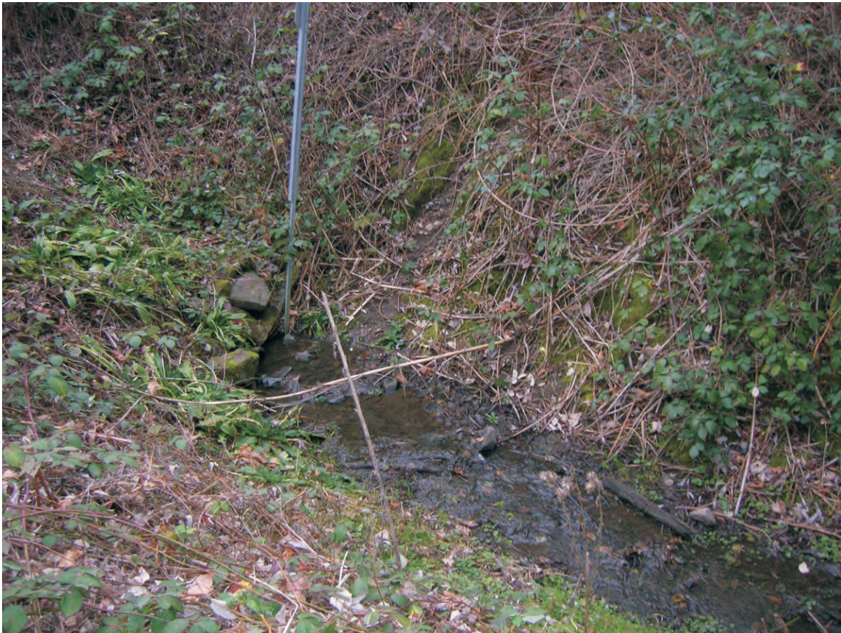
Photo 1. Crystal Creek culvert outlet. View is south.
