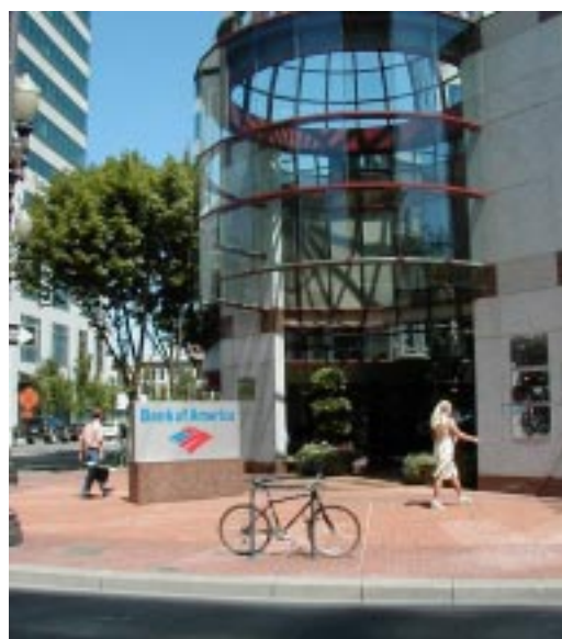
Not Recommended: "Suburban-styled" monument signs at building entries (Second and Morrison, Portland)
