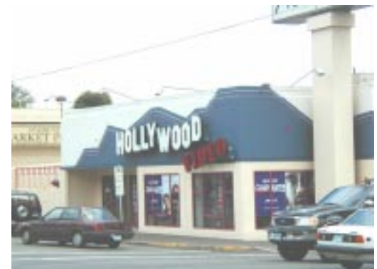
Not Recommended: Building facades designed primarily to serve as a sign (NW 20th and Burnside, Portland)
