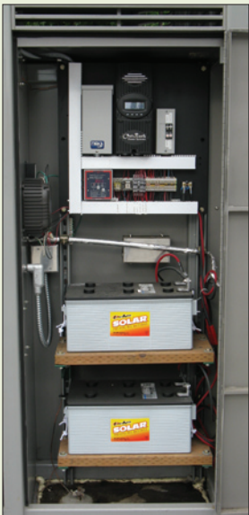
Solar mechanics accessed through rear panel
