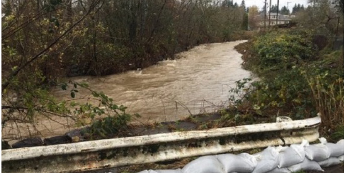
Sandbags Line Johnson Creek during 2015 Flooding
