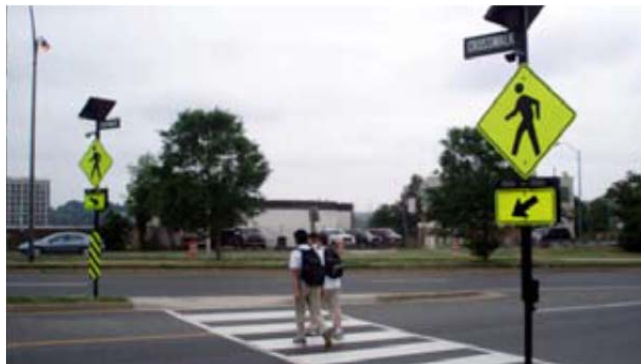
Rectangular rapid flash beacon and median island
