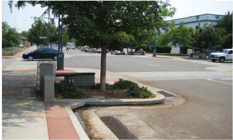
Curb extension with landscaping
