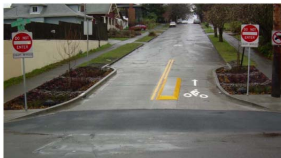
Intersection with semi-diverter, curb extension, and green street features. Source: City of Portland.
