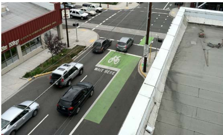
Figure 16. Bicycle boxes improve active transportation on many streets in the Central Eastside Industrial District. Similar transportation improvements could improve multi-modal access and circulation within the Study Area.
