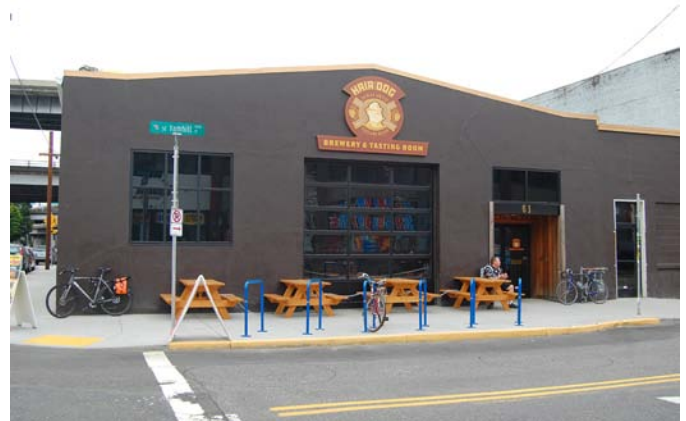
Figure 7. Warehouses easily convert to more active light manufacturing facilities such as a brewpub and tasting room.
