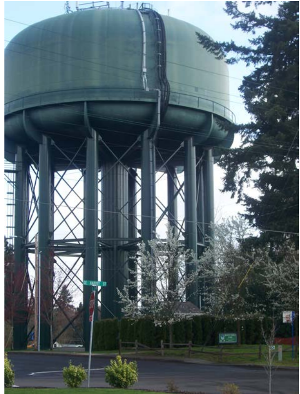
Figure 3-6. Elevated Reservoir
