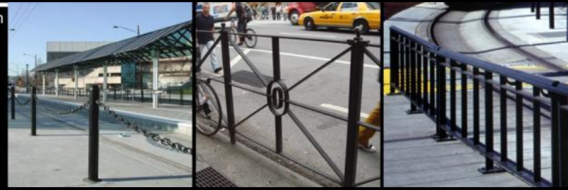
Pedestrian Barriers / Railing
