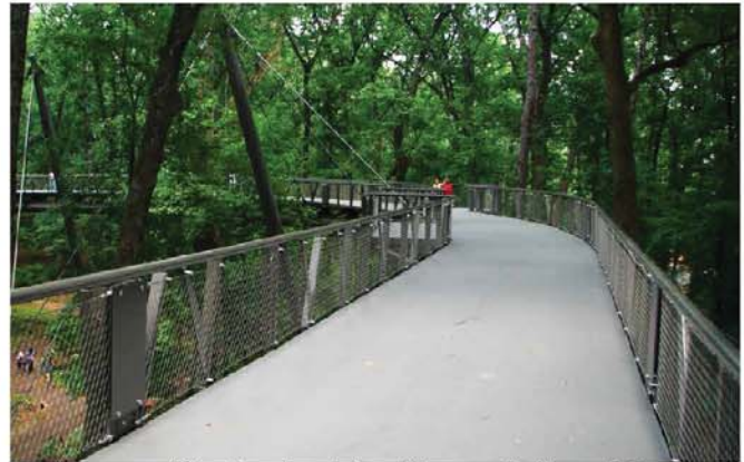
12' wide elevated multi-use path through the forest
