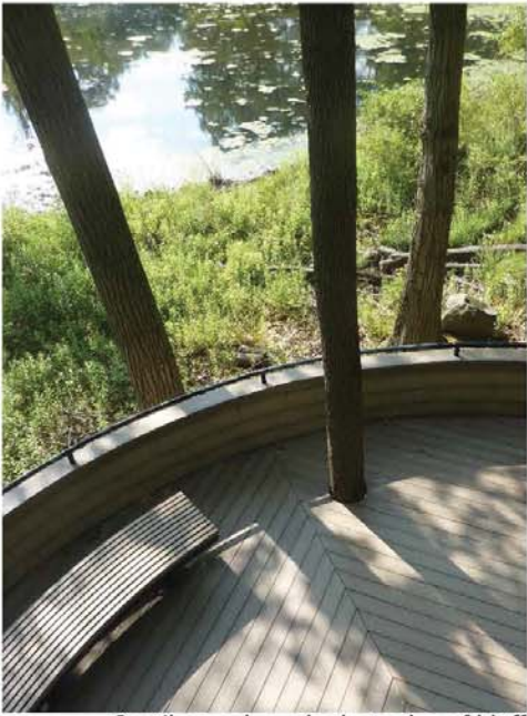
Cantilevered overlook at edge of bluff
