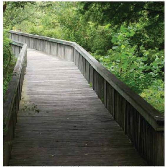
Cantilevered boardwalk/multi-use path at McLoughlin
