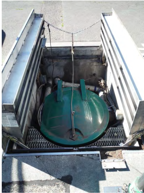
Figure 3.2 – Traffic-Rated Cover for Dry Well Access Hatch
