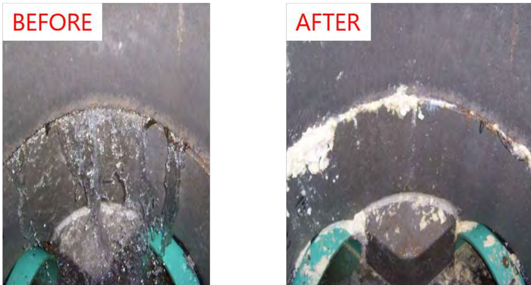
Figure 3.7 – Resin Injection Performance (Source: Resiplast US Inc.)
