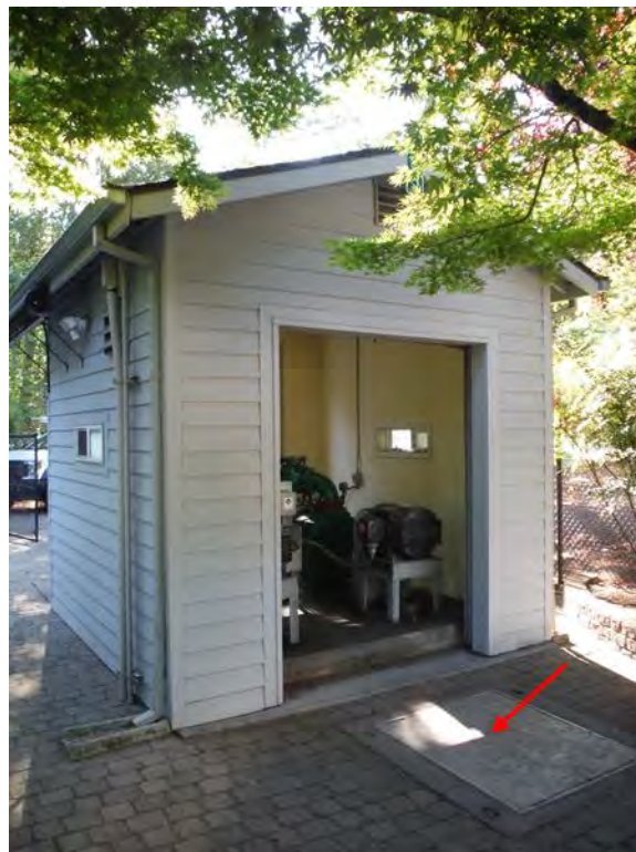
Figure 3.23 – Flowmeter Vault Access Hatch
