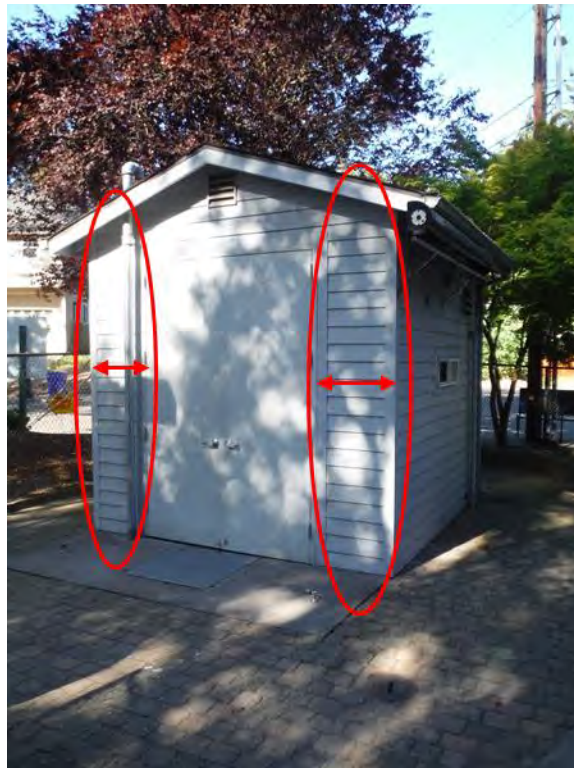
Figure 3.27 – Narrow Vertical Piers of Shear Wall
