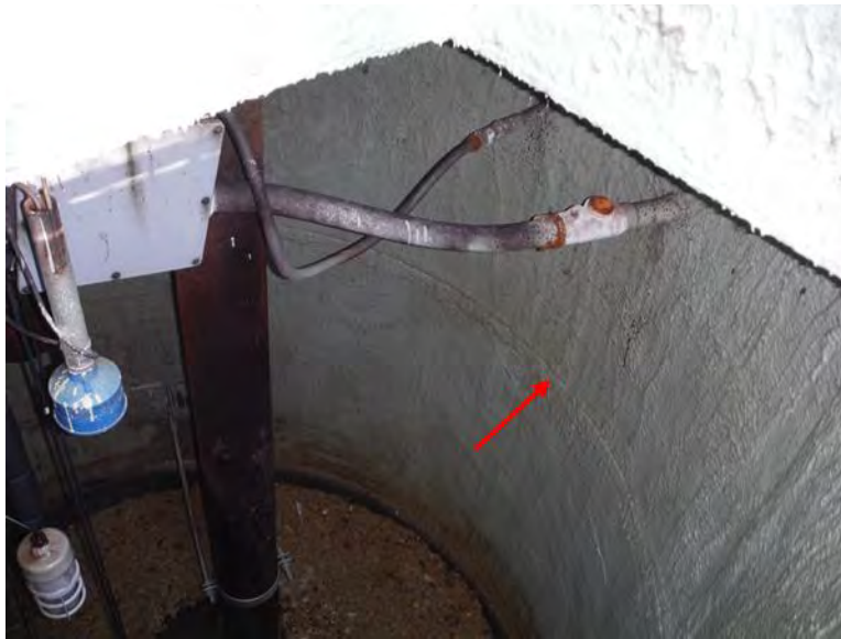
Figure 3.25 – Precast Concrete Wet Well Joint between Adjacent Stacked Riser Sections
