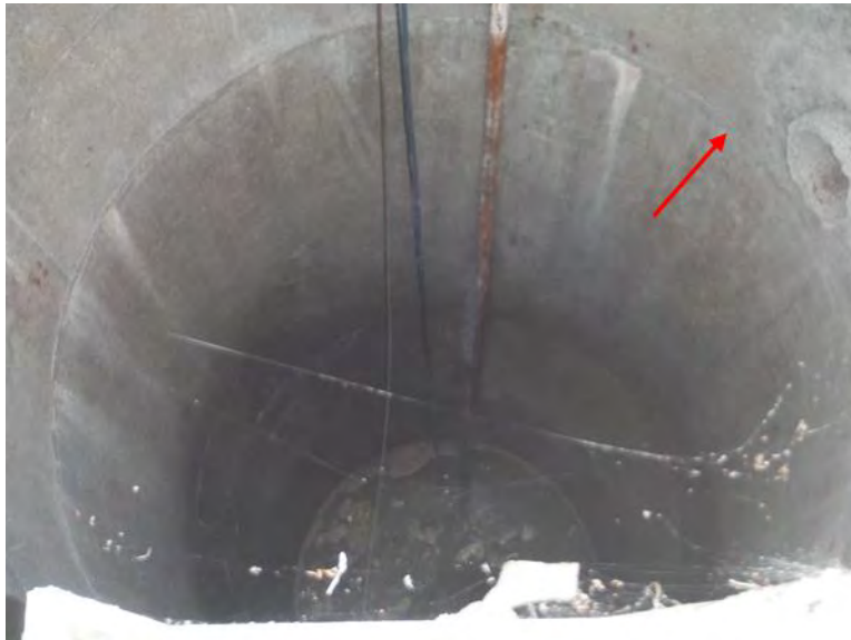
Figure 3.4 – Precast Concrete Wet Well Joint between Adjacent Stacked Riser Sections
