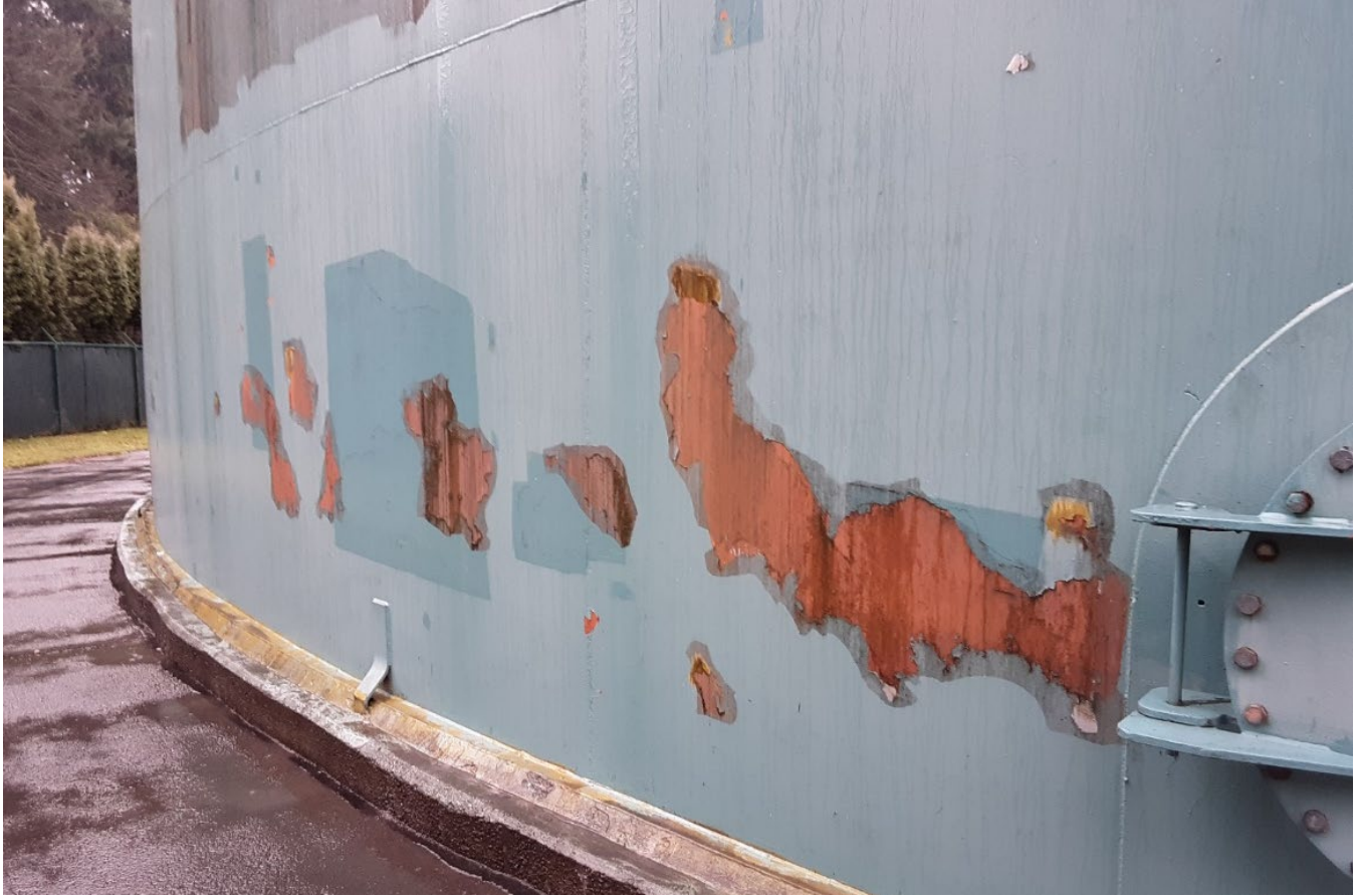
Figure 2-1. Stanley Reservoir Exterior Paint Condition
