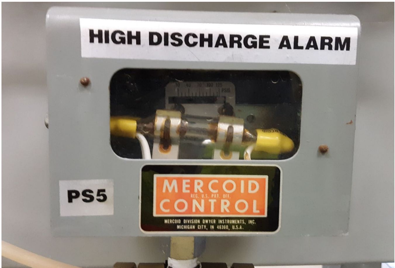
Figure 2-4. Mercury Switch
