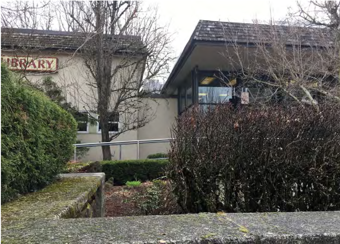
5. Looking east at the c.1906 volume (left) and the 1997 enclosed entry vestibule (right)
