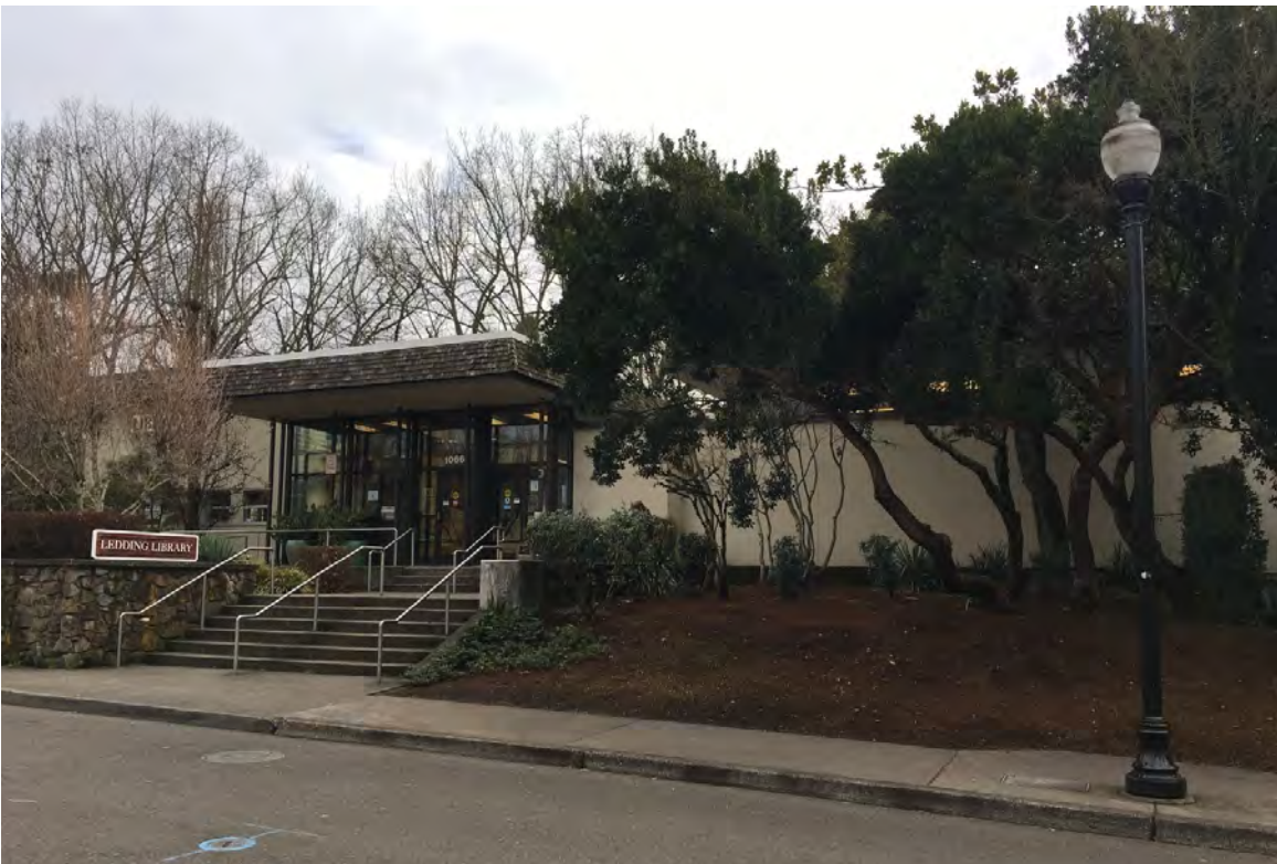
4. Primary entry on the west side of the building
