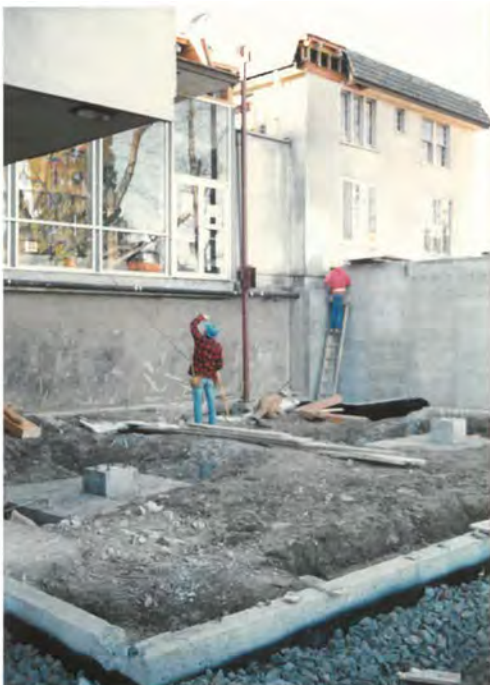
16. 1986 construction photo looking northwest
