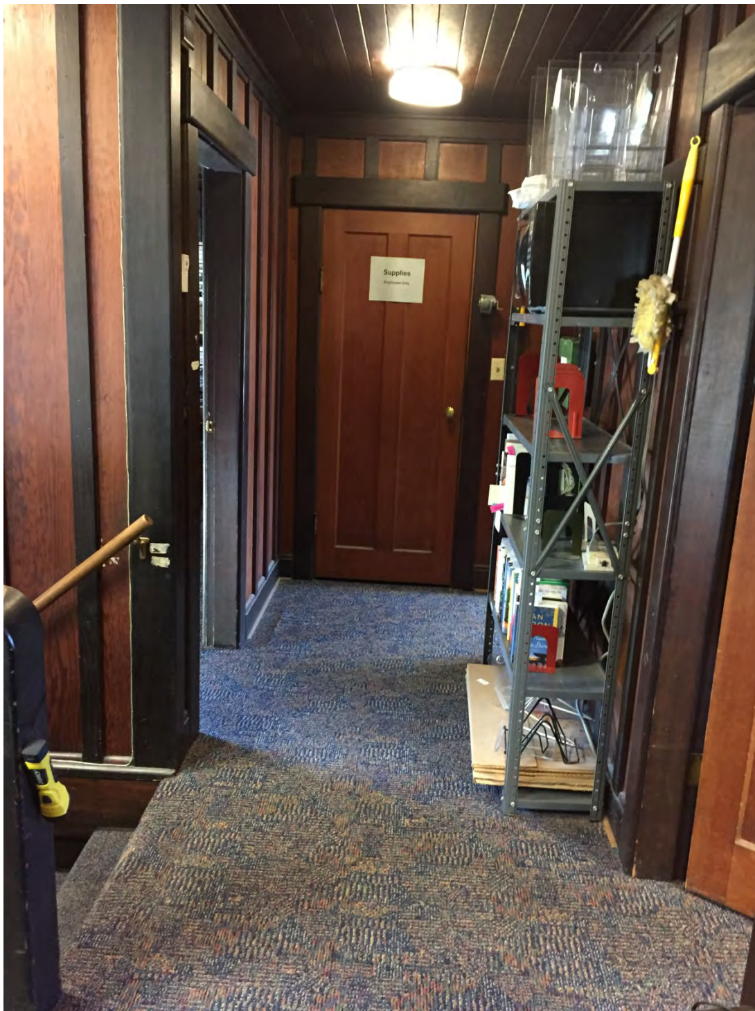
13. Interior, upper level of c1906 structure, looking west
