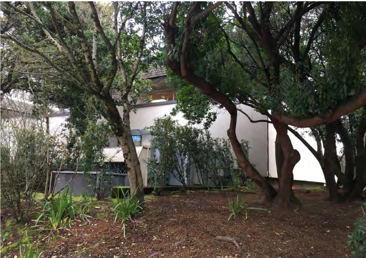
6. Southwest corner of the building
