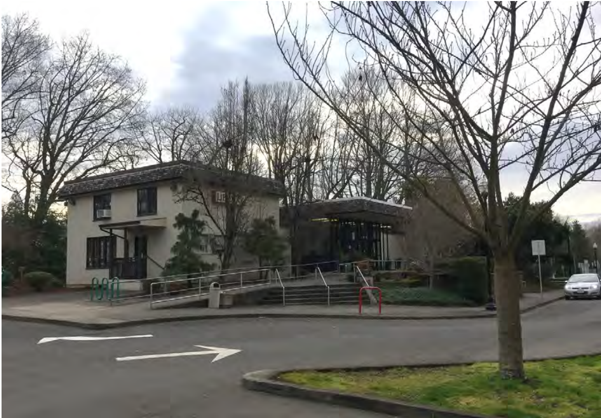
1. Northwest corner of the building
