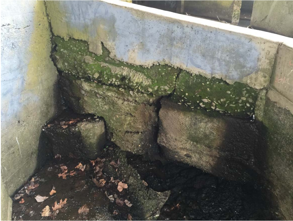
Looking East – Fish Ladder Weir in Foreground
