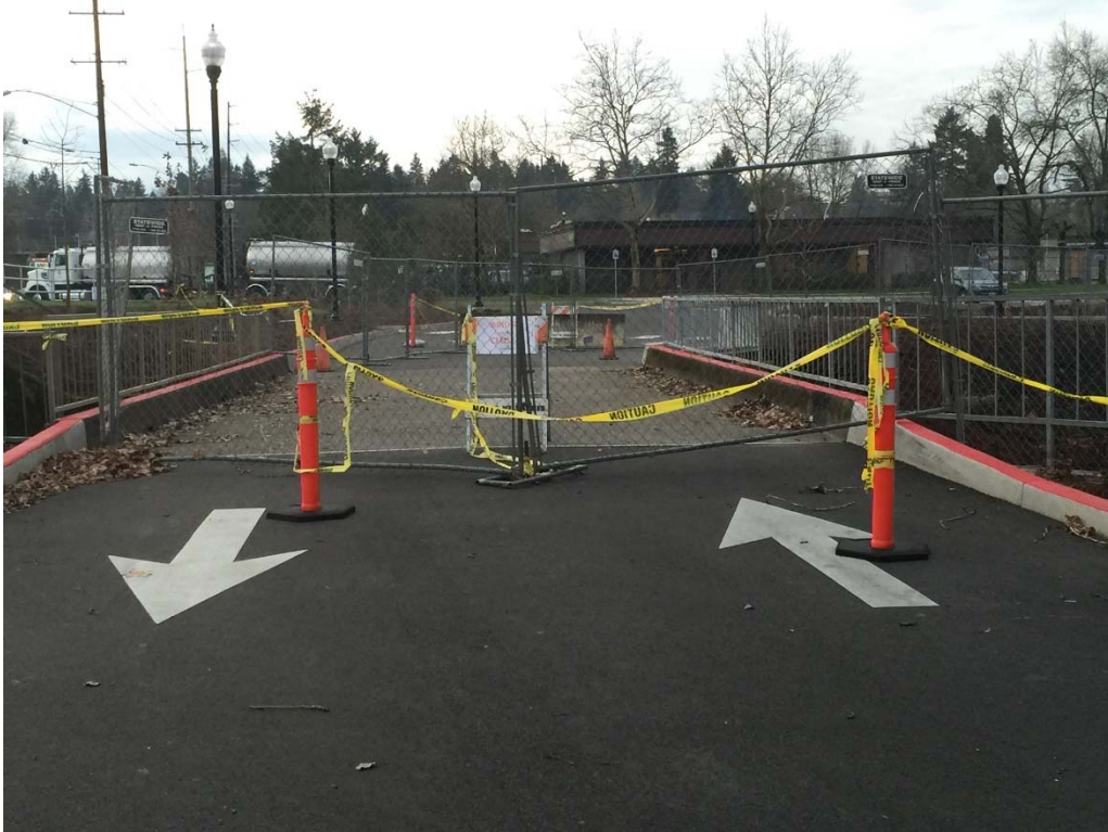
Looking South from the North Across the Bridge
