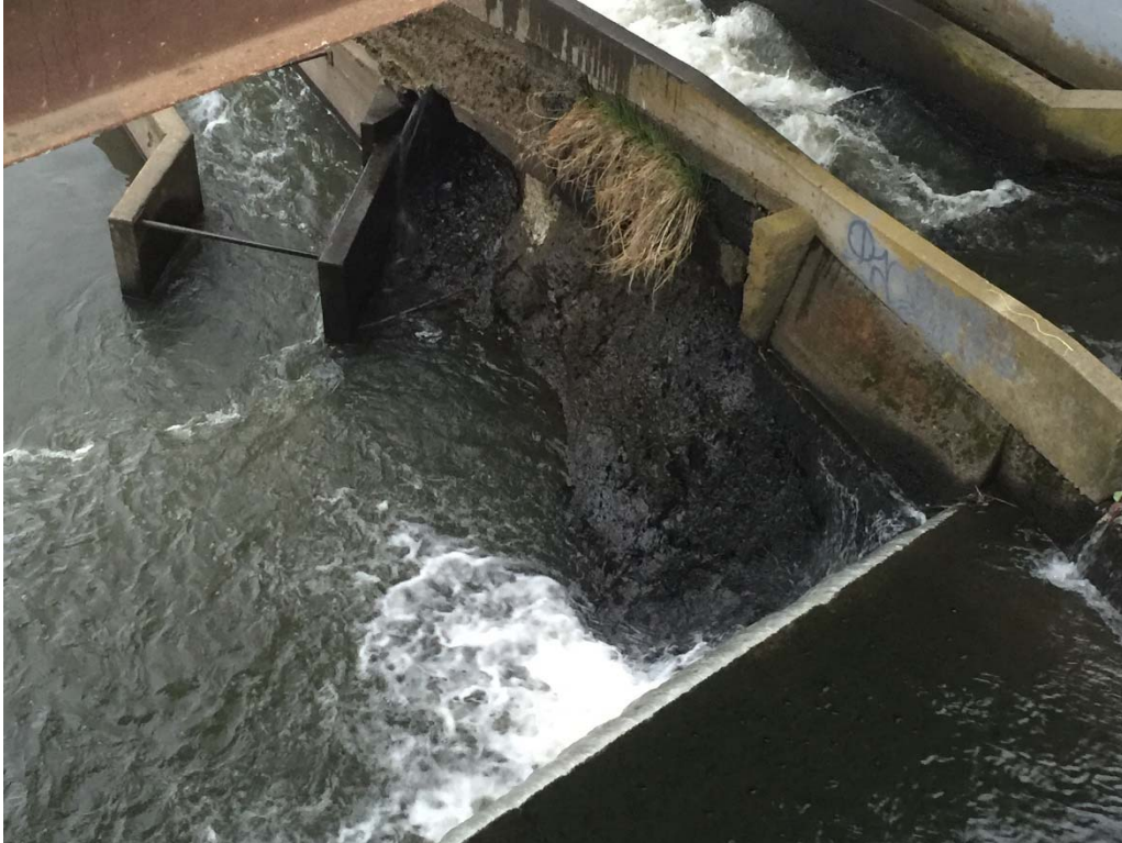
Looking North at Fish Ladder
