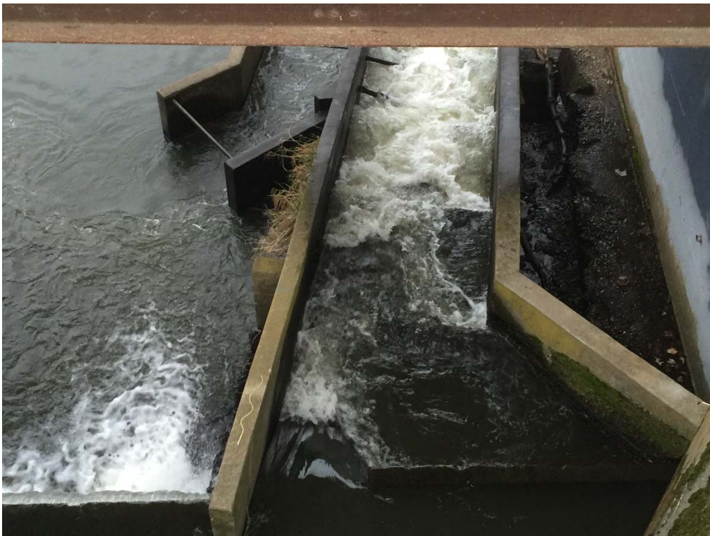
Looking West – Fish Ladder and North Abutment
