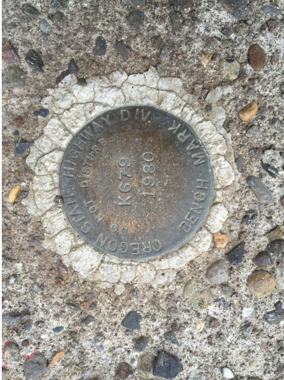
Survey Marker, South Abutment, West Wingwall
