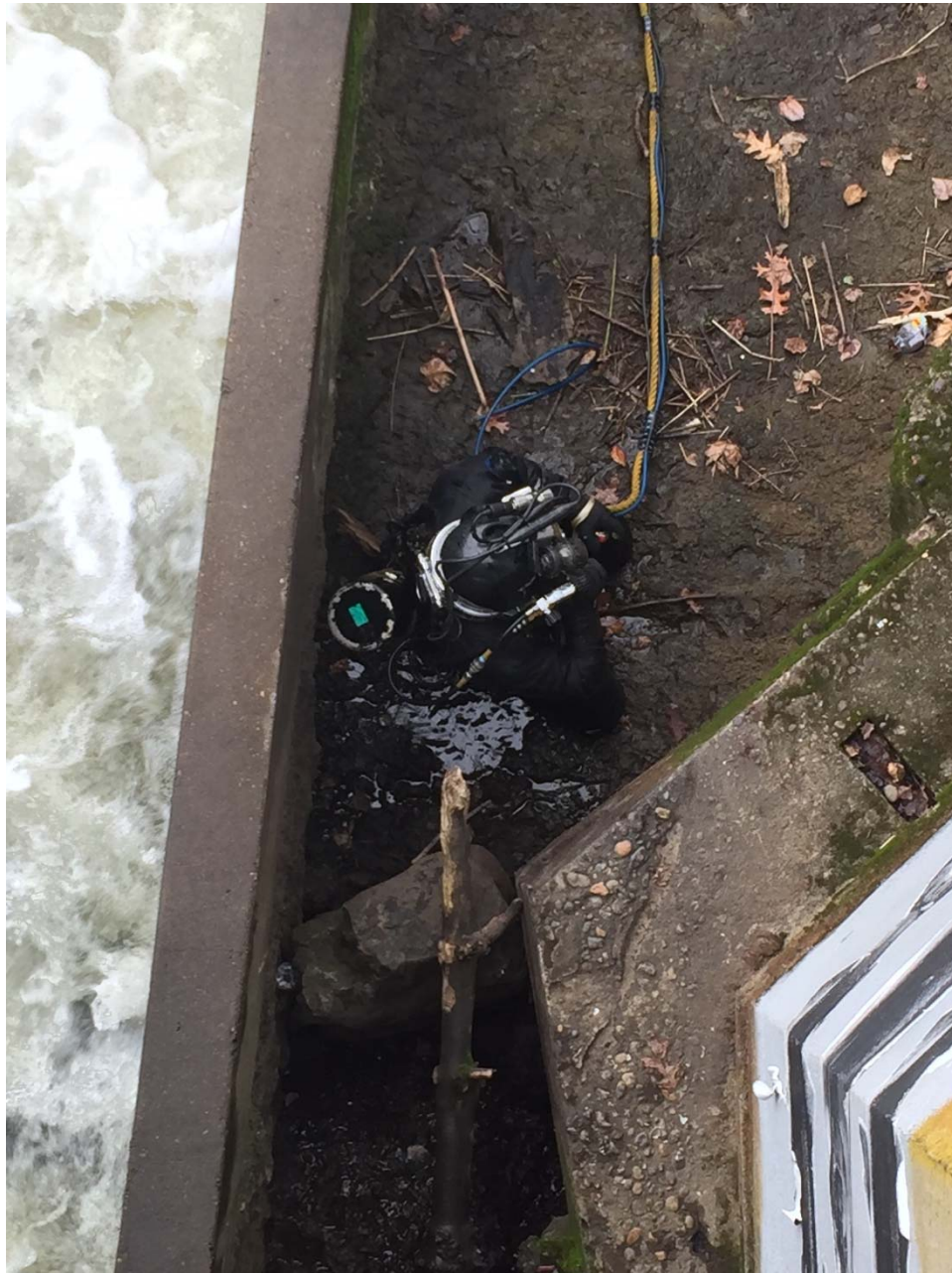
Looking at North Abutment SW Corner
