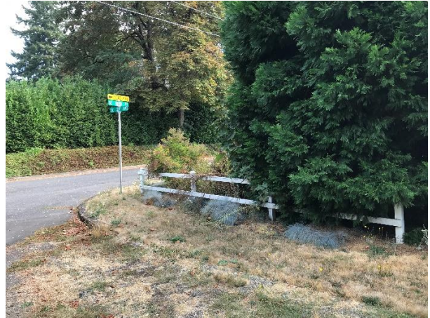
Photo 4: Shrubs restricting sight distance
