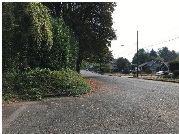
Photo 2: Condition of vegetation near intersections and street lights
