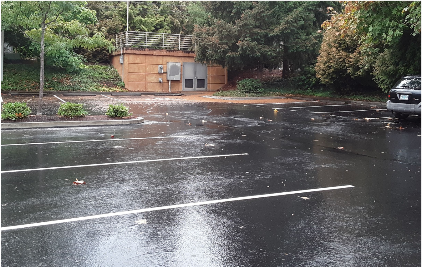
Figure 2-5. Lava Drive Pump Station Parking Lot
