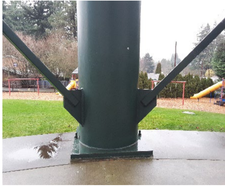
Figure 8-2. Tower Base Plate
