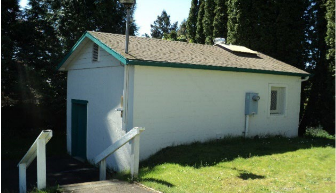
Figure 8-4. Well No. 3 Pumphouse
