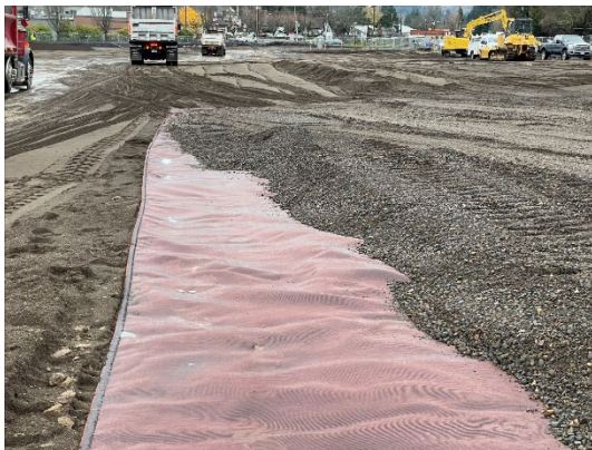
11/19/21 Parcel 1 grading. Mirafi fabric shown underneath import pavement rock.
