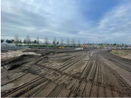
11/10/21 Parcel 1 fill placement. View to southwest from the center of Parcel 1.
